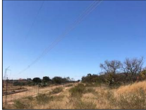
Figure 31 – P: existing powerline adjacent to game fence (facing north).
