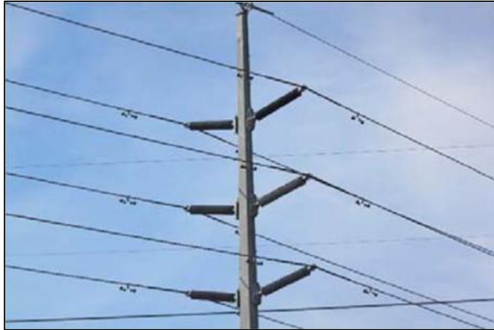
Figure 6 - View of a typical single steel pole (monopole) structure.
