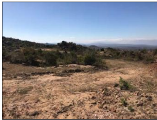
Figure 24 – J: Slope erosion on Quayle farm.
