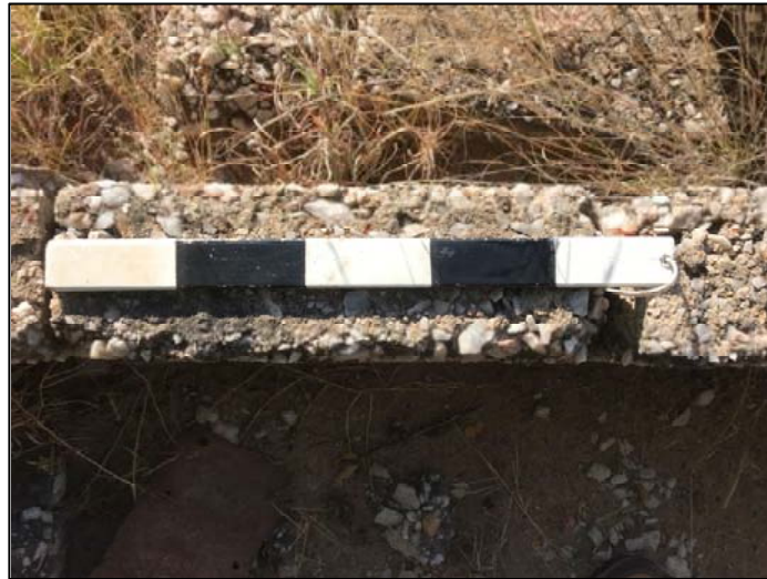
Figure 76 - Views of the foundation at NT12.
