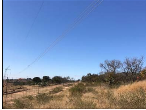
Figure 31 – P: existing powerline adjacent to game fence (facing north).
