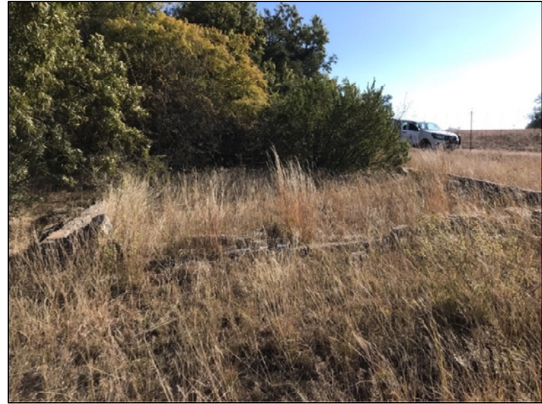
Figure 51 – View of the foundation at NT12.
