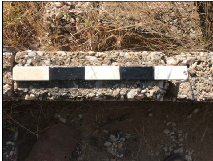
Figure 76 - Views of the foundation at NT12.
