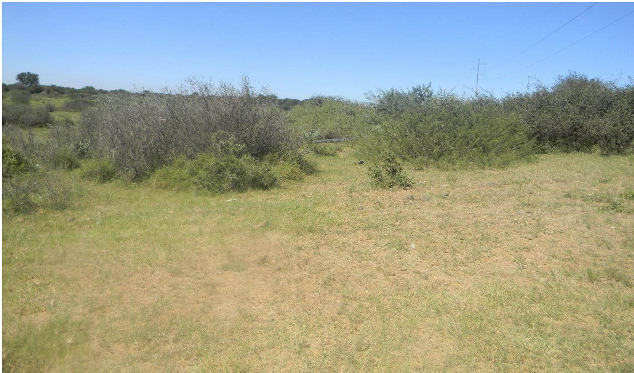
Figure 20: View of powerline route along existing 132kv line
