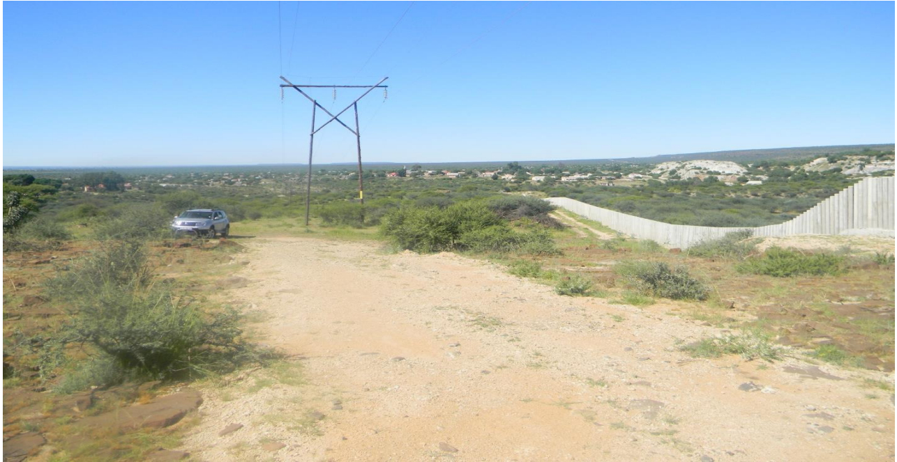
Figure 17: 66kv powerline running close to the site boundary
