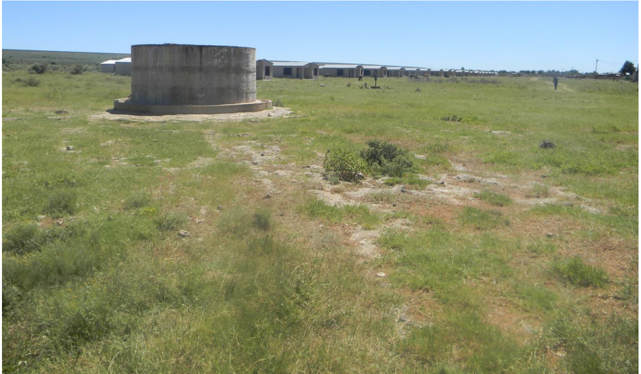
Figure 21: View of some residential developments in the project area
