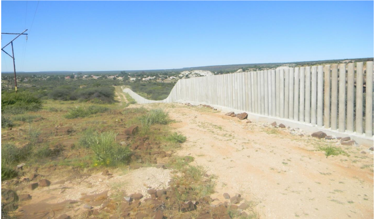
Figure 15: Existing 22kv powerline running near the site boundary.
