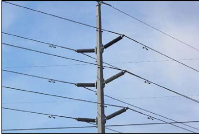
Figure 5 - View of a typical single steel pole (monopole) structure.
