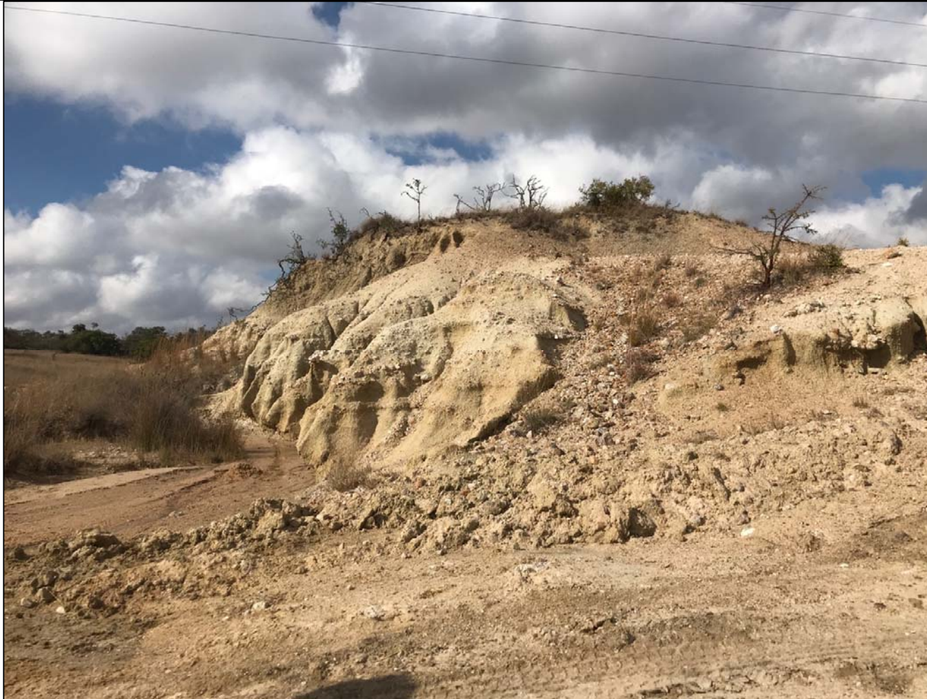
Figure 40 - View of the gully erosion at WP04.
