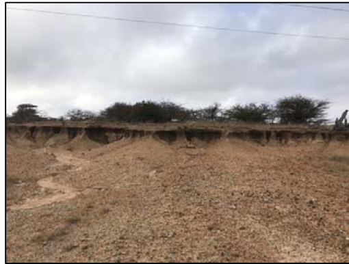
Figure 18 – L: Erosional gully.
