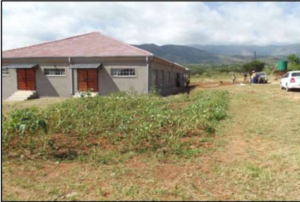
Figure 7. The site on 1 April 2015. Note that the excavation had been filled again.
