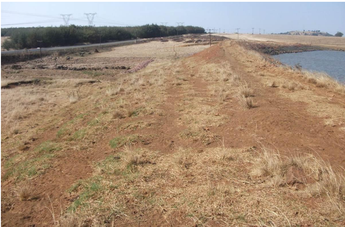
Figure 6: View across dam wall looking southwards
