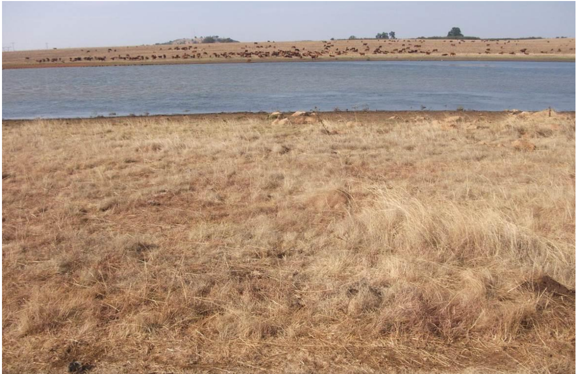
Figure 7: Northern side of dam looking southwards
