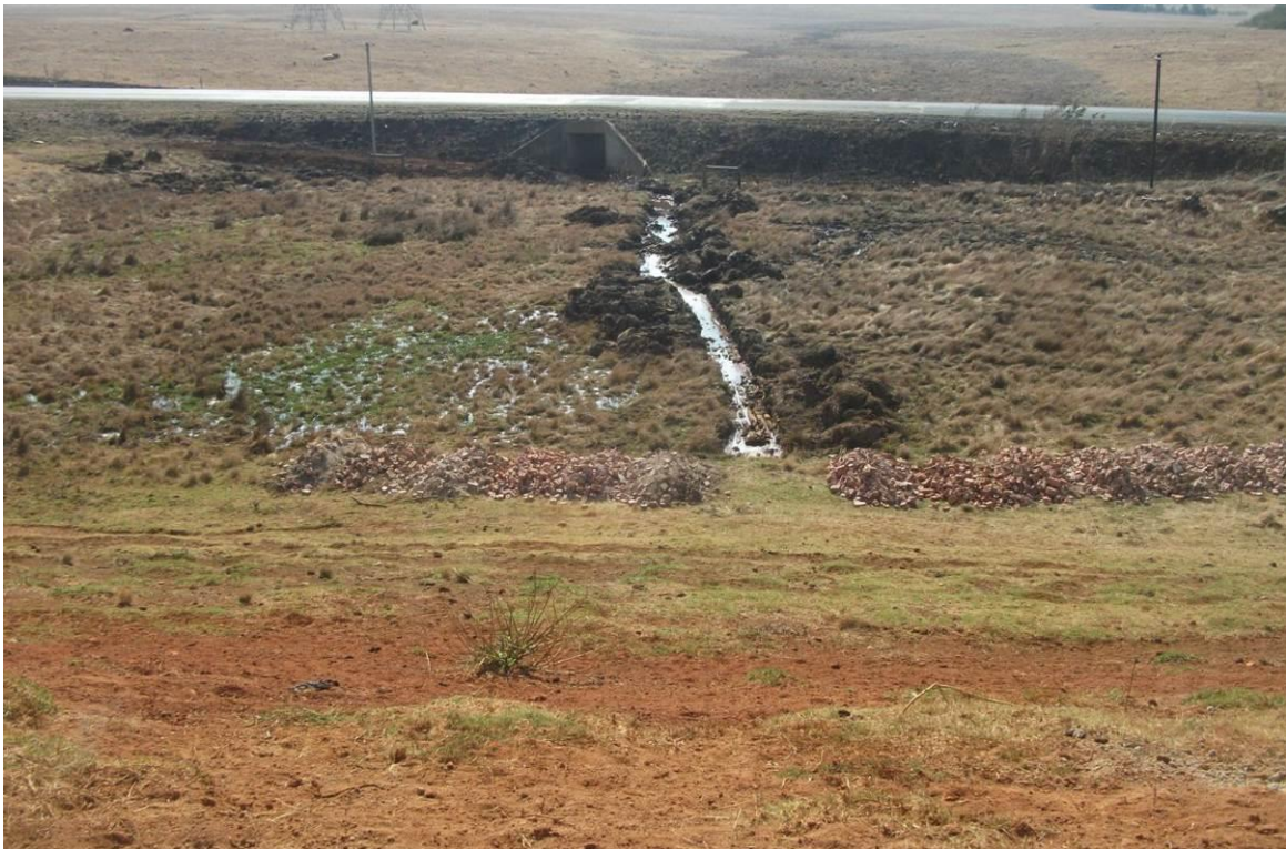
Figure 5: Wetland with channel to divert water towards culvert
