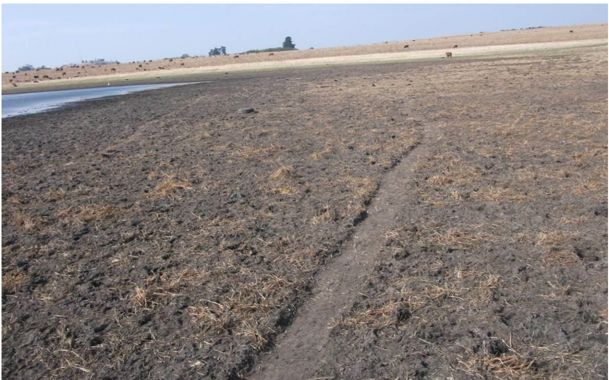
Figure 10: Western end where stream enters dam
