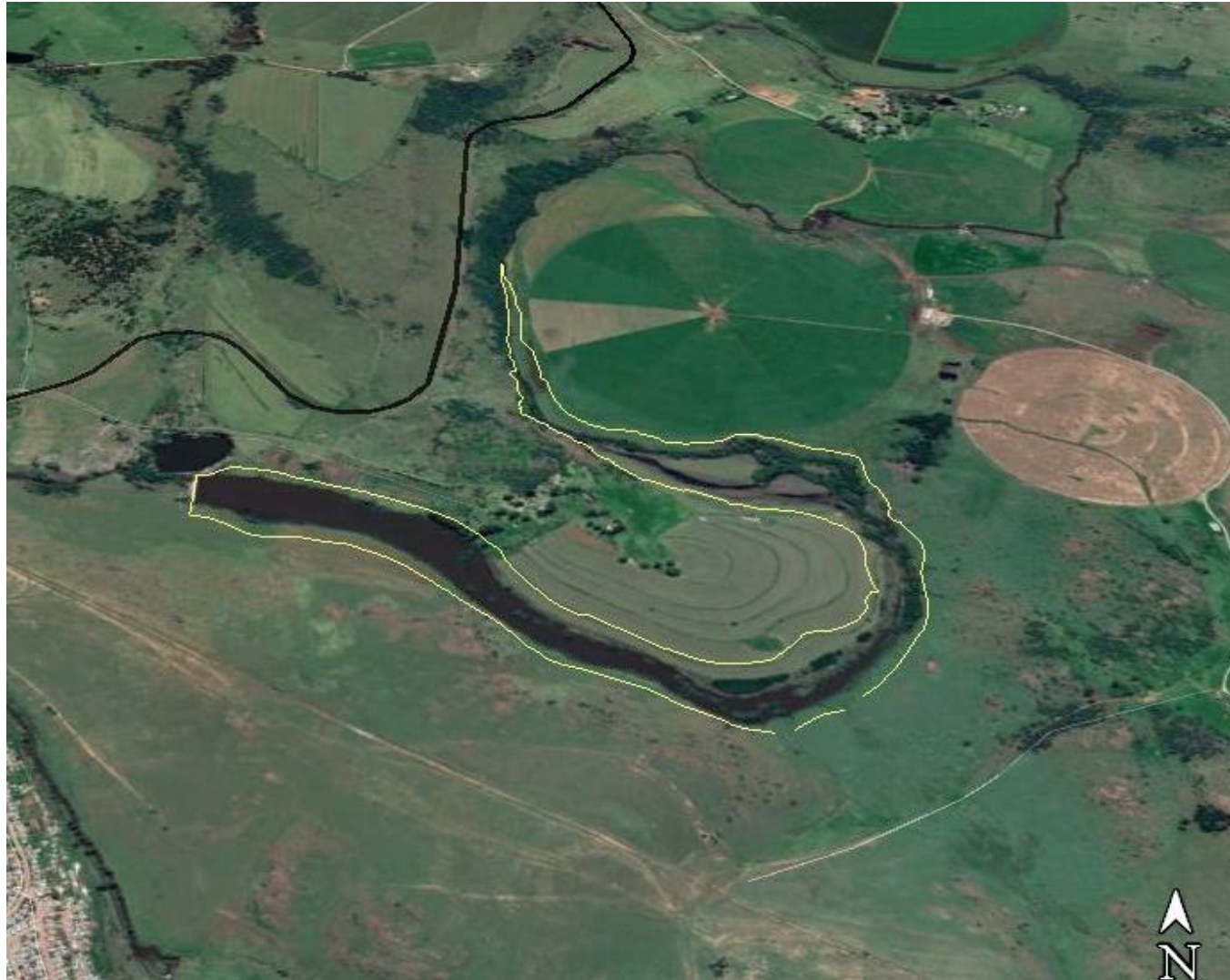
Figure 2: View of dam and proposed expansion
