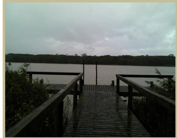
BOARD WALKS AND JETTY DUE FOR UPGRADE
