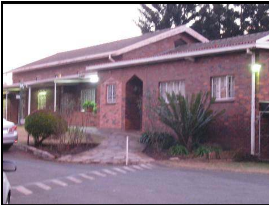
Figure 10. Main Building at the Alan Wilson Shellhouse and Bowling Greens
