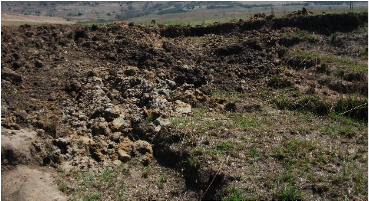
Figure 7: Excavation work on western side of river
