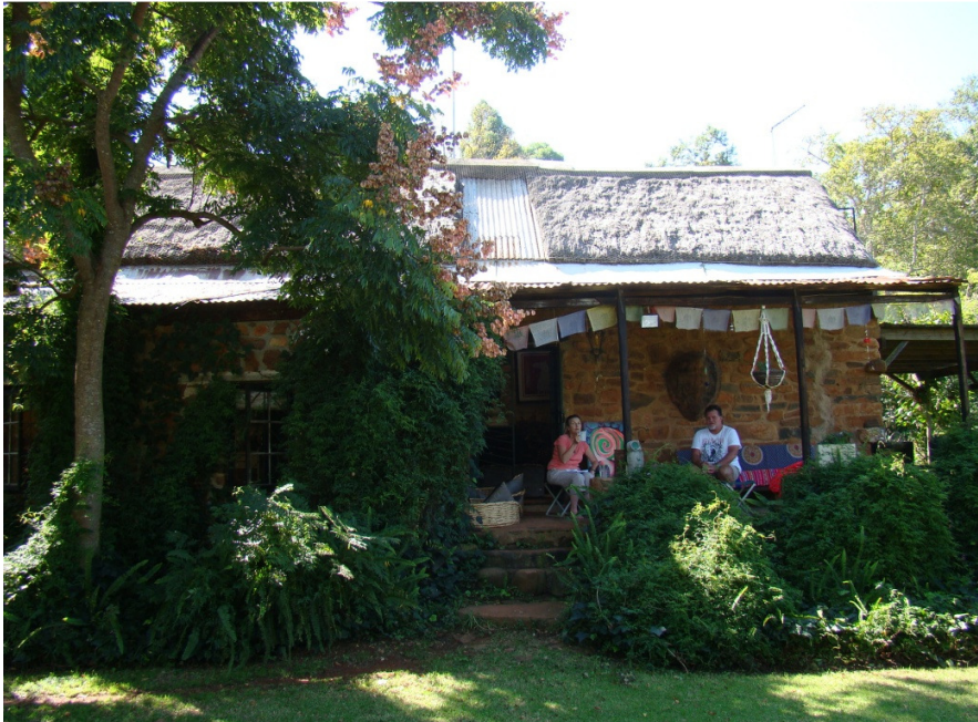
Fig. 5: Existing house on Stand 3.
