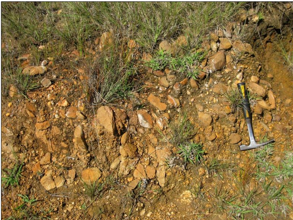
Fig. 24. Section through typical colluvial deposits exposed in dam excavation showing poorly-sorted clasts of Table Mountain sandstone in a sandy to silty matrix (Hammer = 32 cm) (Loc. 442).
