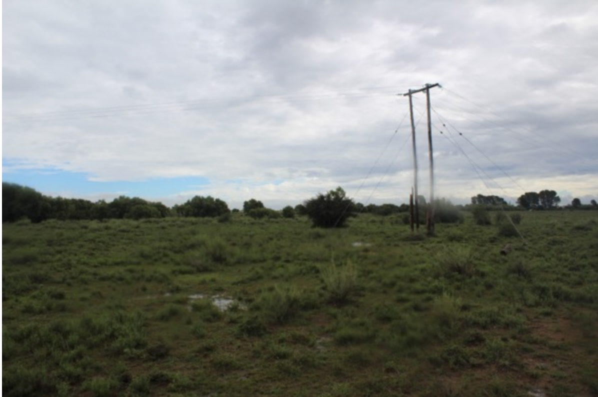
Figure 6- Existing powerline that the interconnection line it will connect to
