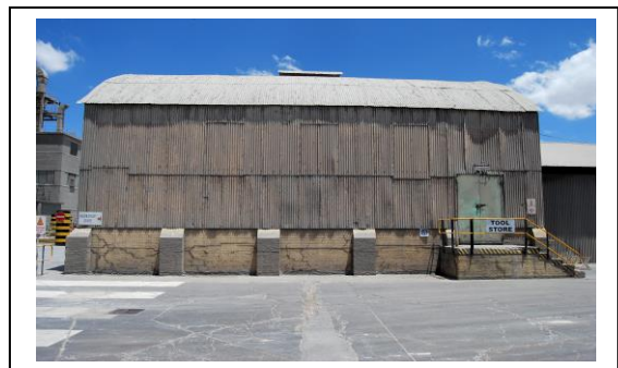
Fig. 34 View looking south
