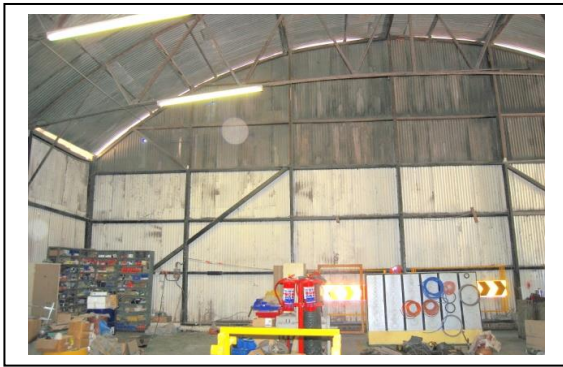
Fig. 16 View looking to south-west corner.
