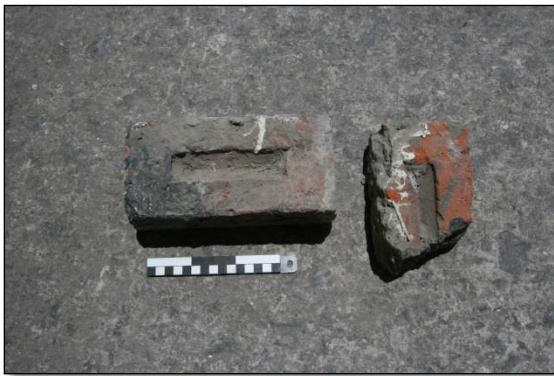
Fig. 4 Handmade bricks used in the foundation walling.
