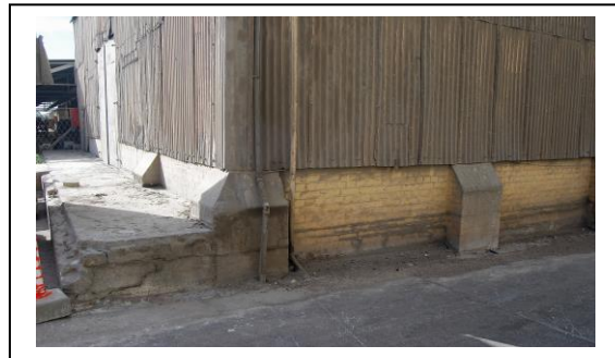
Fig. 38 buttresses on south-east corner
