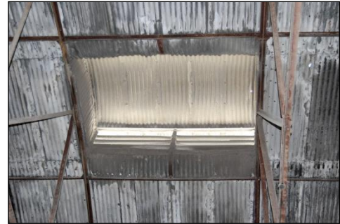
Fig. 9 View of the air vent from the building.
