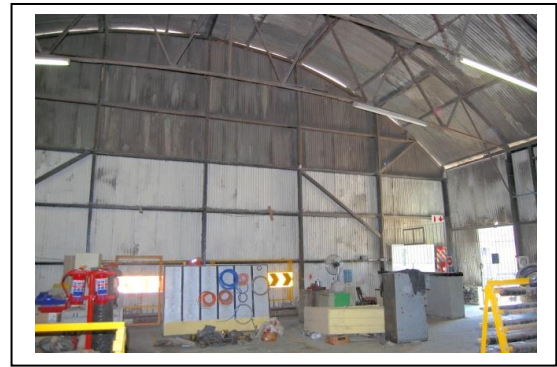
Fig. 17 View looking to north-west corner.
