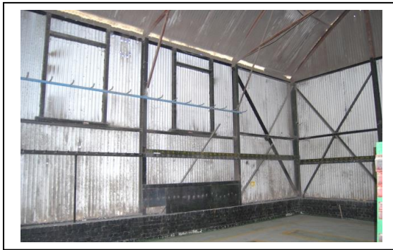
Fig. 20 North-east corner, note the bund wall.
