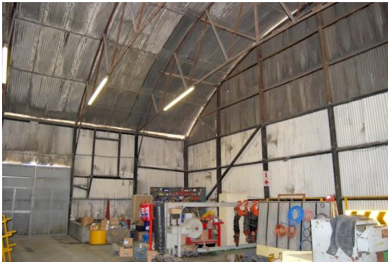
Fig. 11 View of the timber structure gable end looking south-west.
