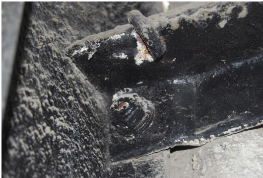
Fig. 5 Single bolt connection of a girt.
