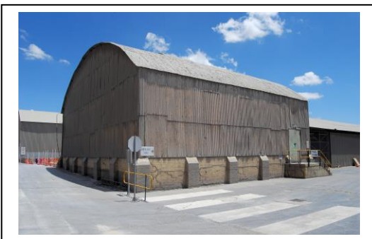
Fig. 33 View looking south-west
