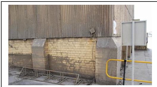
Fig. 39 Buttresses on the north-east corner.
