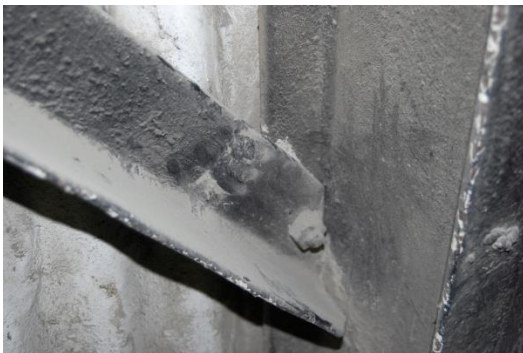
Fig. 7 Single bolt connection of a cross-brace.
