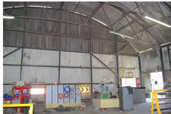
Fig. 12 View of the timber structure gable end looking north-west.
