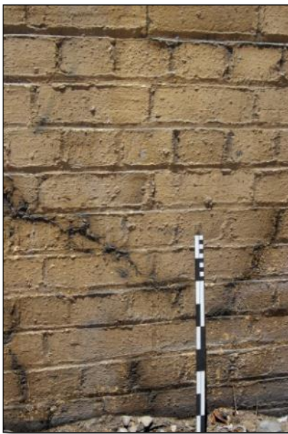
Fig. 3 External wall showing brickwork in English bond.
