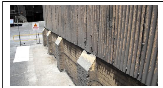
Fig. 40 Buttresses on the north wall.
