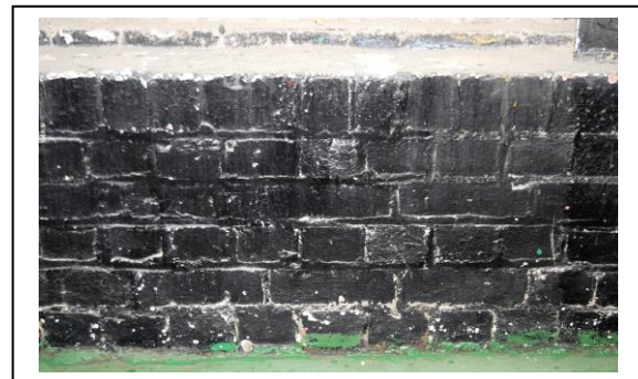
Fig. 25 English bond brickwork on the internal bund wall.
