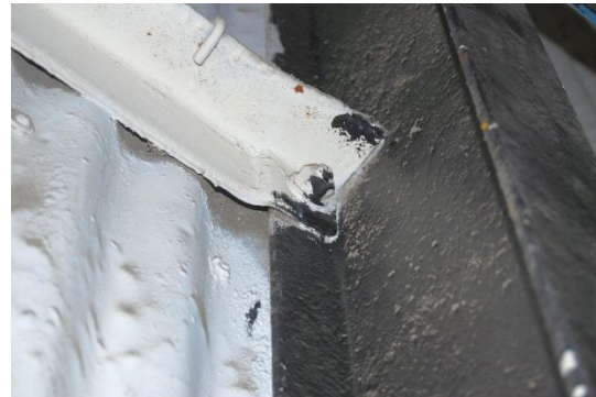
Fig. 6 Single bolt connection of a girt.
