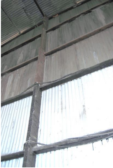
Fig. 13 One of the main timber columns with timber girts.
