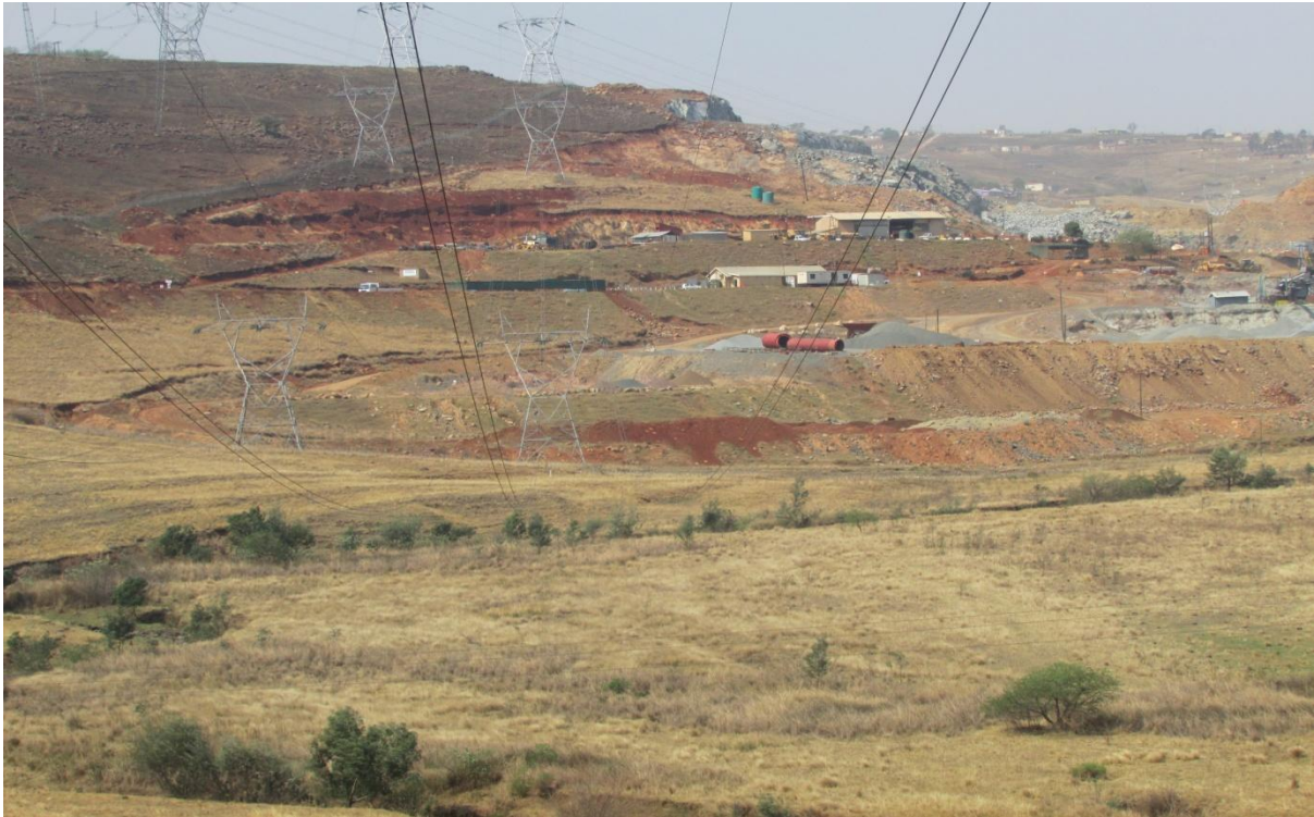
Figure 6: View of the area where the power line will transverse over mining area.
