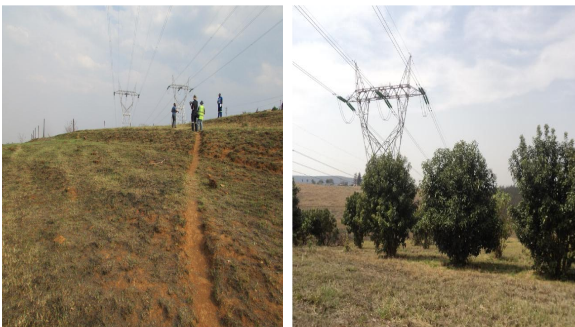
Figure 5: View of some of the area where the power line will transverse.
