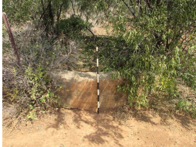
Figure 29: Cement dam at Site 1.
