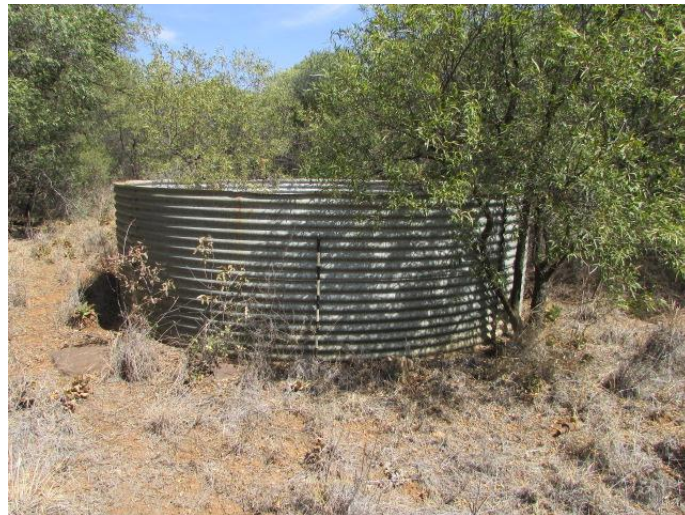
Figure 30: Corrugated iron & cement dam close to Site1.
