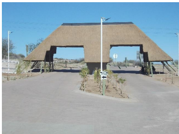
6(a) Existing thatched roof entrance to resort development
