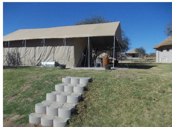
6(b) Existing tented chalets on development
