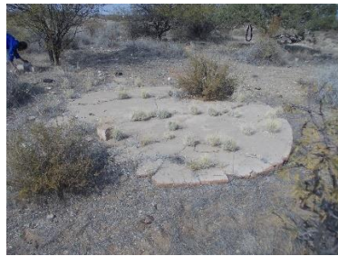
18(a) Cement foundations
