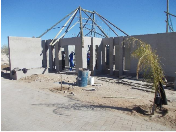
6(c) Construction on site at time of our study
