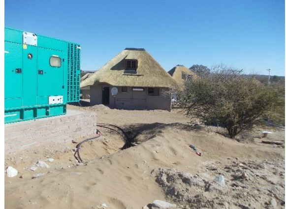
6(d) Construction on site with generator
