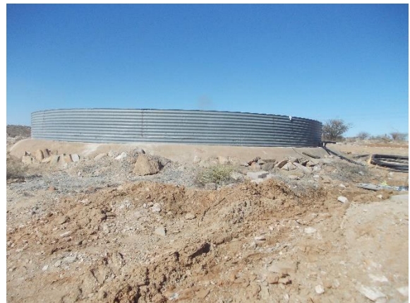
6(f) Reservoir on site adjacent to waterworks/supply
