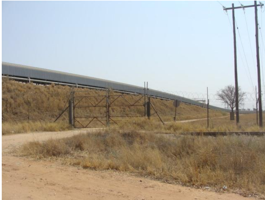
Figure 9: Overland conveyor close to one of the surveyed routes on the farm Hanglip.
