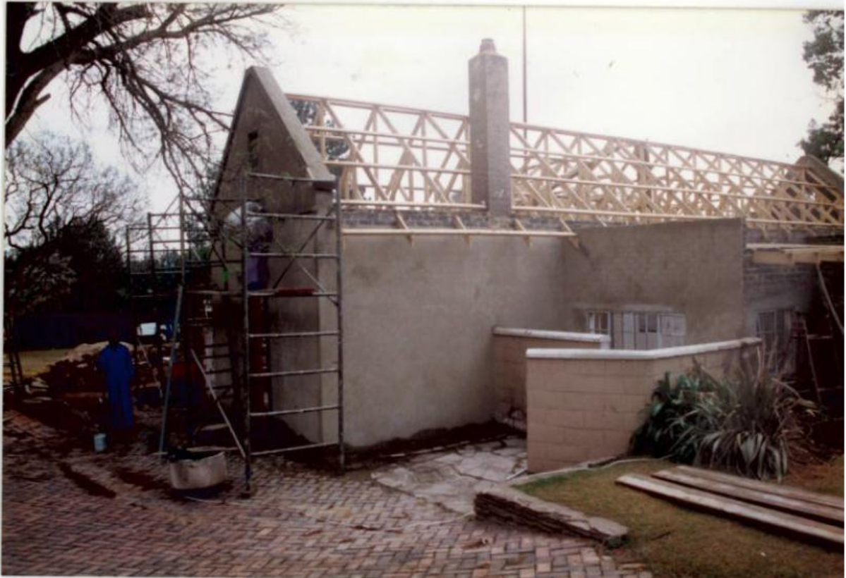
Figure 24: House being rebuilt.
