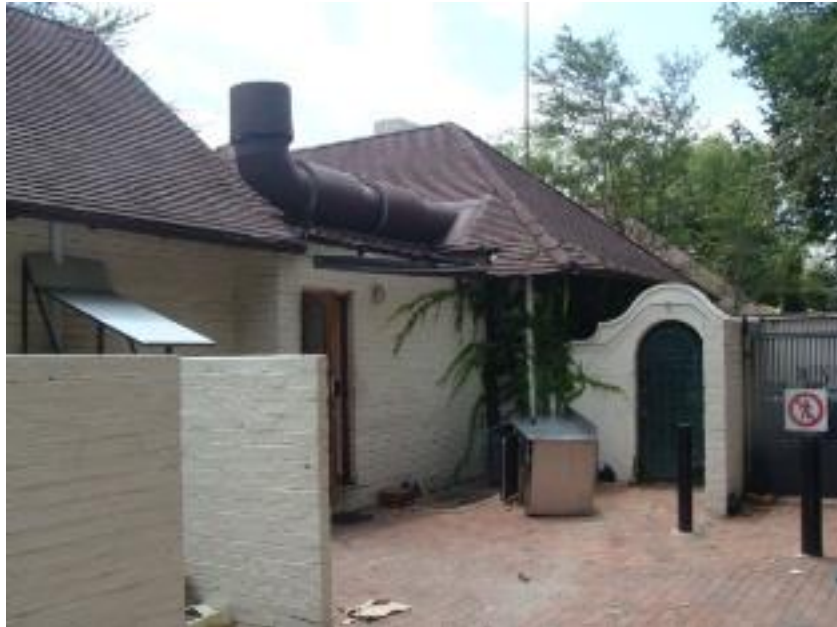
Figure 17: Back view of restaurant/house.
