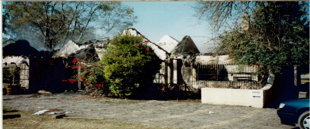
Figure 23: More images showing the extensive damage done by the fire.
