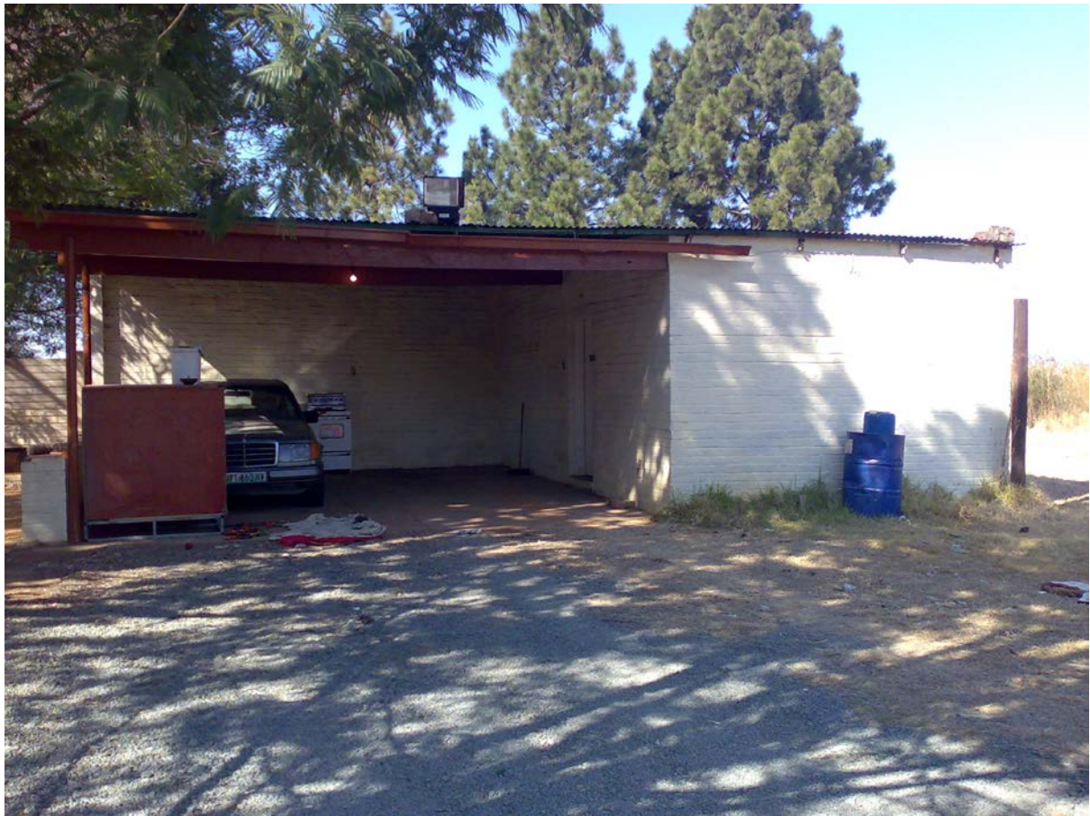
Figure 6: An outbuilding adjacent to the house.
