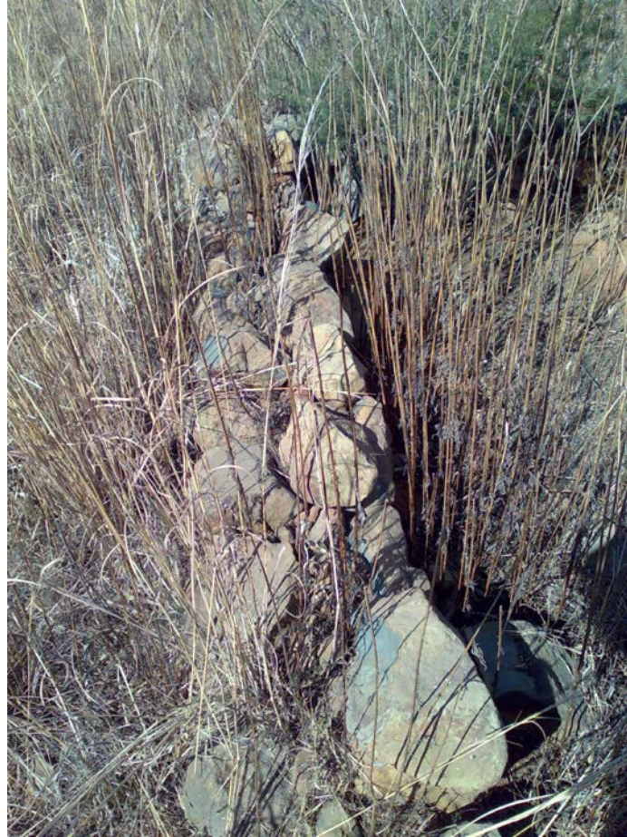
Figure 12: A section of the foundation walling of a house.
