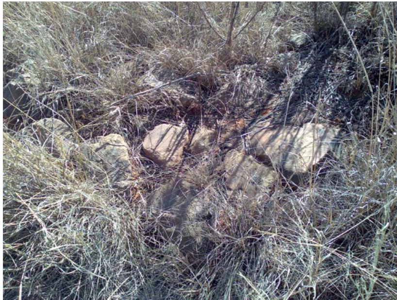
Figure 10: A section of the foundation of one of the houses.
