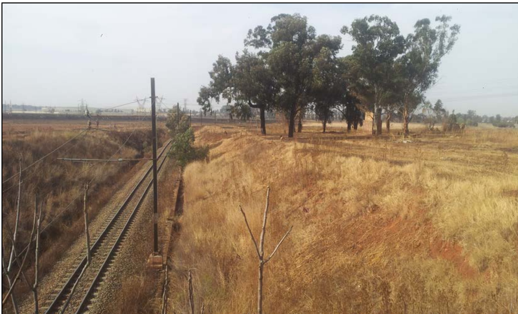
Figure 8: General view of area at the mid-section of the pipeline (intersecting railway tracks and roads)
