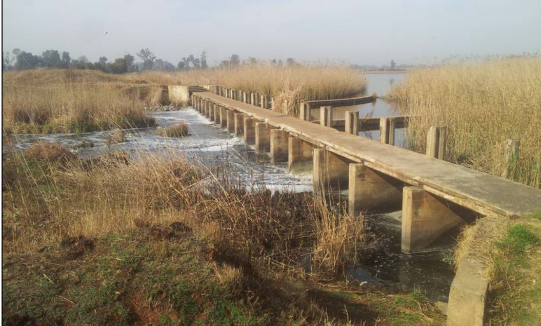
Figure 7: Structures associated with the Cowles Dam
