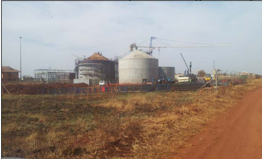
Figure 9: Eastern end of pipeline at the water treatment works plant
