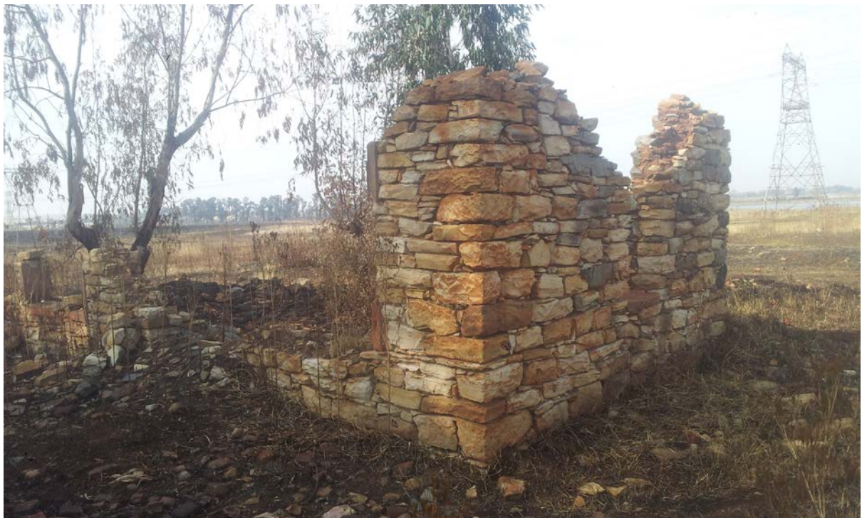
Figure 18: Detail view of the dressed stone work of the house
