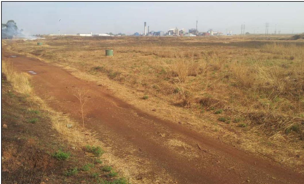
Figure 6: General view of the western section of the proposed pipeline (entering Sappi) (also note the existing pipeline's concrete access shafts)
