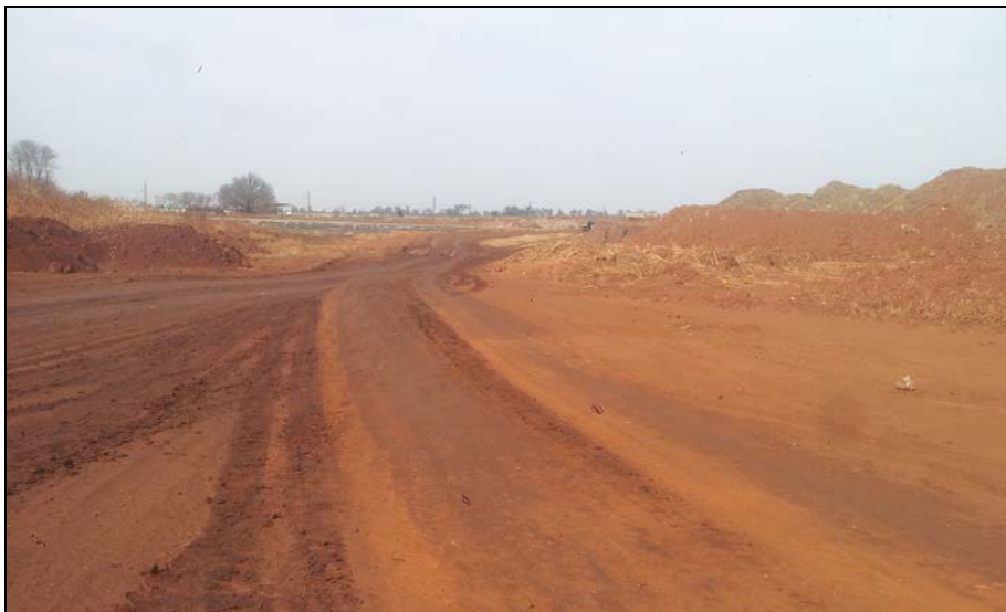
Figure 10: General view of area south of the water treatment works plant
