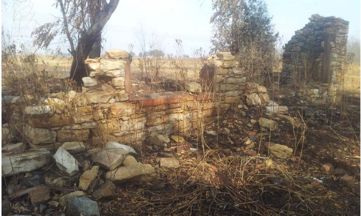
Figure 17: Detail view of the north-facing wall of the house
