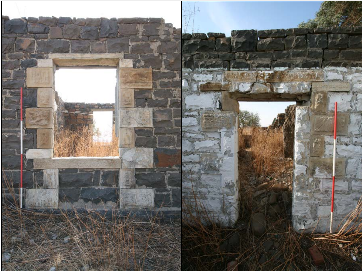
Figure 23: The original back door on the eastern façade of the house was converted into a window (left) and the window on the southern side of the house was converted into a doorway
