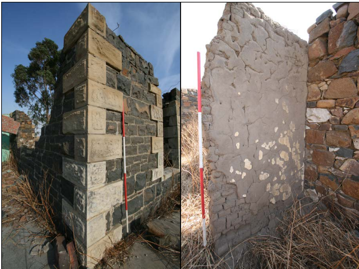
Figure 19: Quoining on the front corner (left) and a section of a sundried mud brick wall inside the house (note white plaster) (right)
