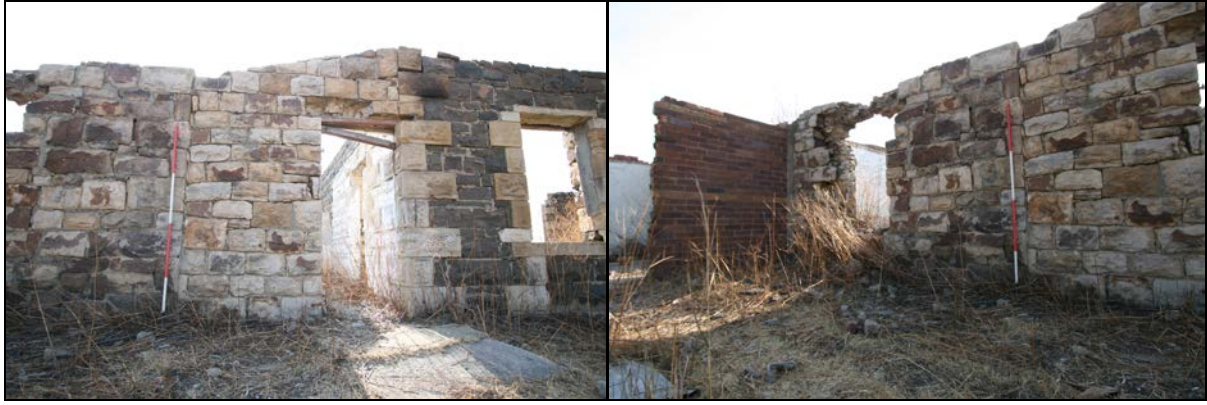
Figure 24: Phase 2 (A & B) is clearly visible on the south facade of the Phase 1 section of the house
