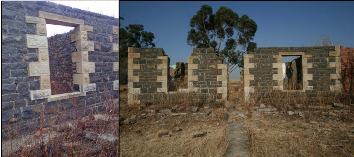
Figure 18: Front façade of the farmhouse (Phase 1) with a detail indicating quoining around a window
