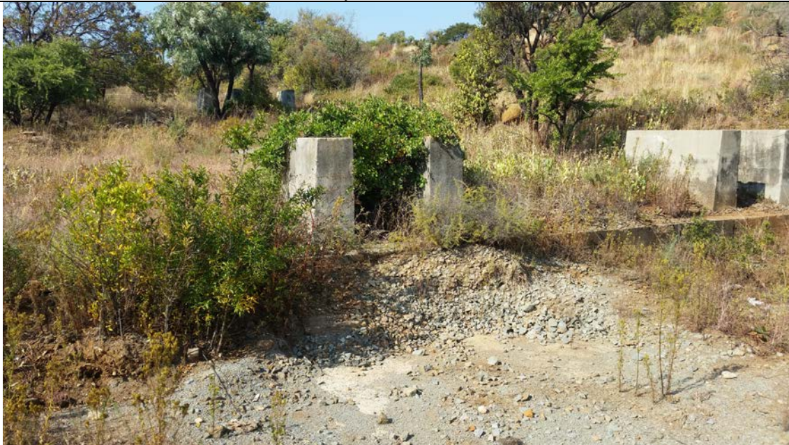
Figure 22: General view of the concrete bases
