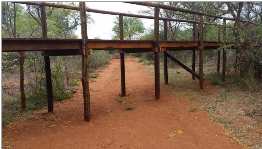
Figure 10: Walkways providing access to the chalets
