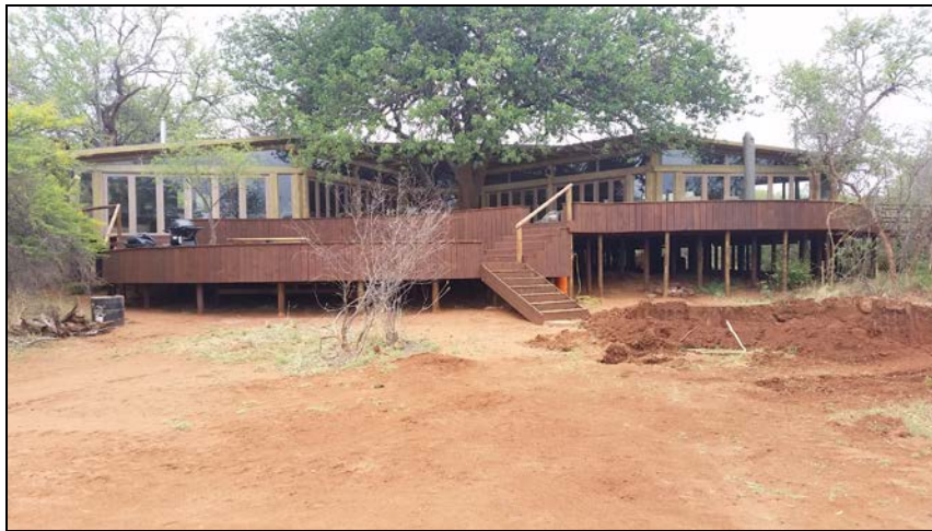
Figure 7: General view of the front of the main lodge structure
