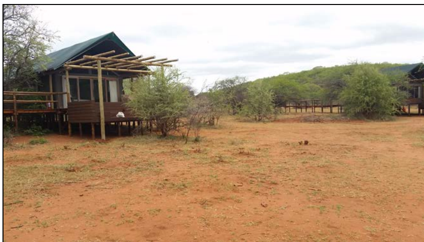
Figure 5: General view of the two four-bed chalets
