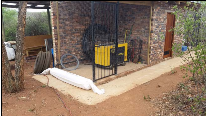
Figure 9: The workshop and generator building
