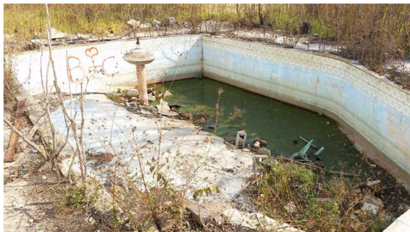
Figure 37: Swimming pool adjacent to the main house
