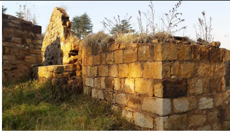
Figure 41: The main structure was built with dressed sandstone and cement
