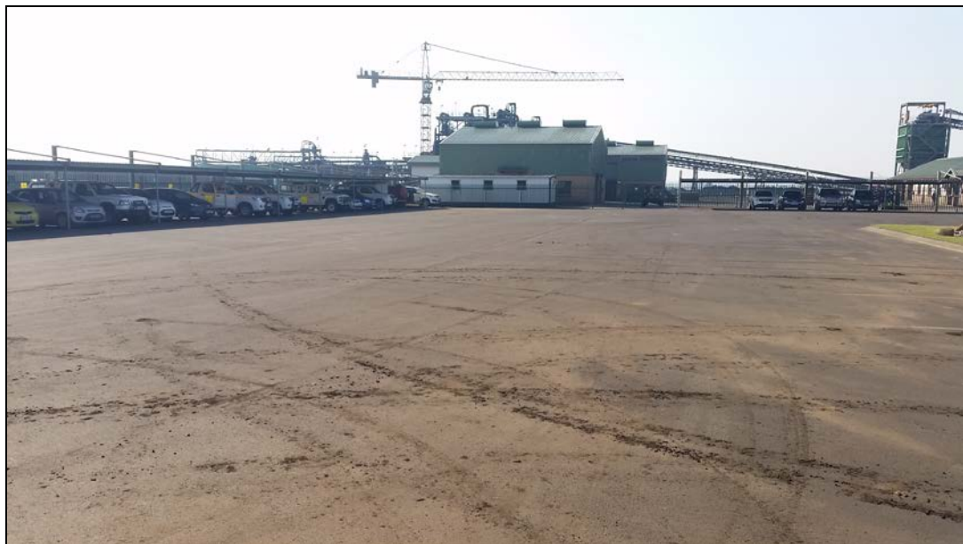
Figure 5: Existing mining infrastructure
