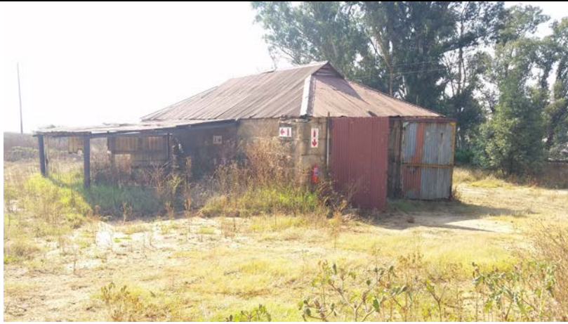
Figure 30: Site 1D: The dressed sandstone shed with corrugated iron roof (additions visible)
