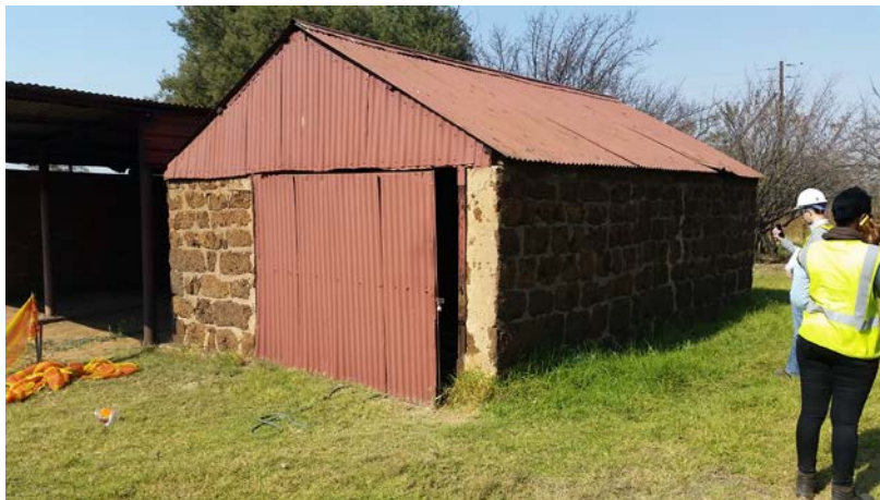
Figure 29: Site 1C: The small square shed with dressed stone and corrugated iron roof
