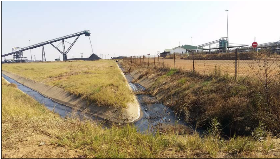
Figure 6: Existing mining infrastructure
