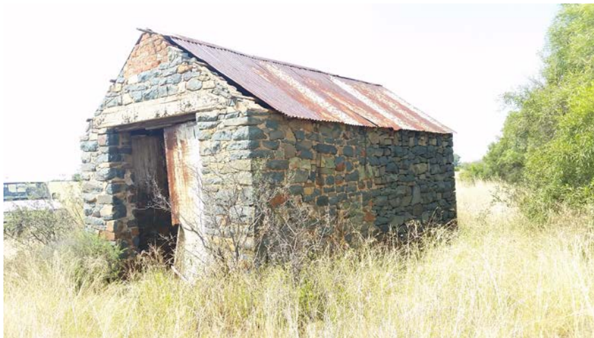
Figure 30: Alternative view of the structure
