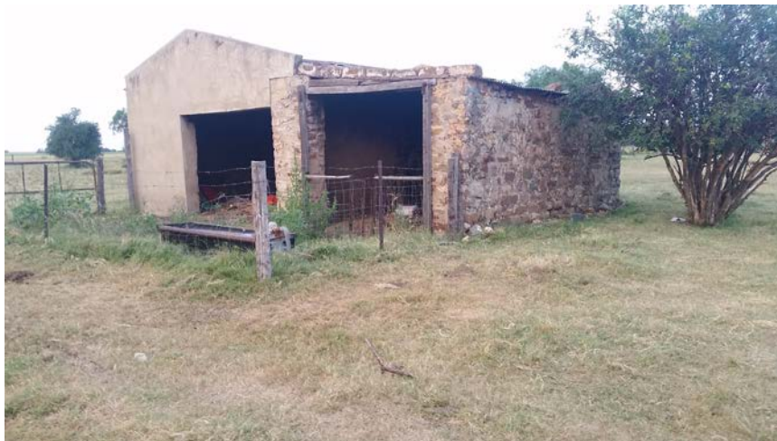
Figure 22: The stone shed with later addition (wooden lintel)
