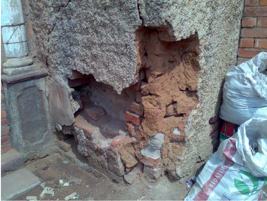
Figure 27: Unstable condition of a section some of the outer walling
