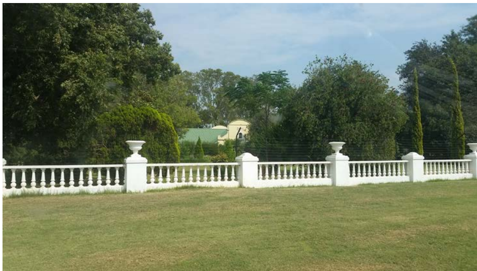
Figure 36: Northern face of the main farmhouse
