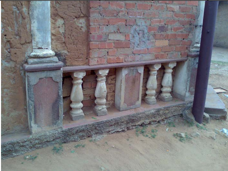
Figure 25: Alterations to the veranda pillars
