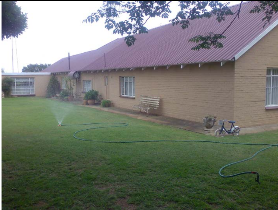
Figure 29: Adjacent farmhouse built in the mid-1940s (notice additions and alterations which continued until recently)
