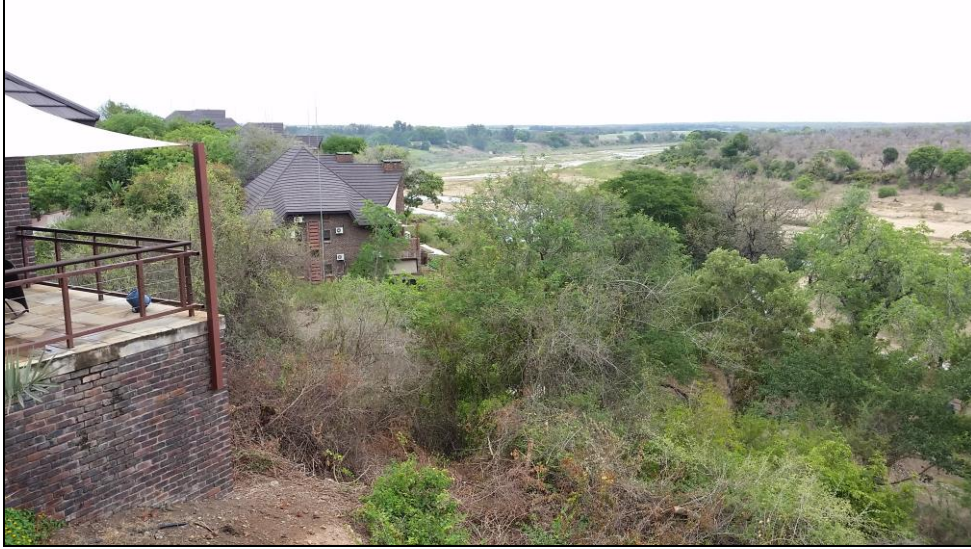
Figure 9: General view of the existing lodge units along the Crocodile River
