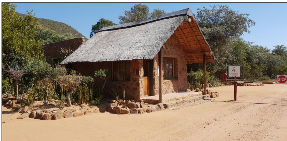
Figure 7: General view of existing infrastructure at South Gate (central section)
