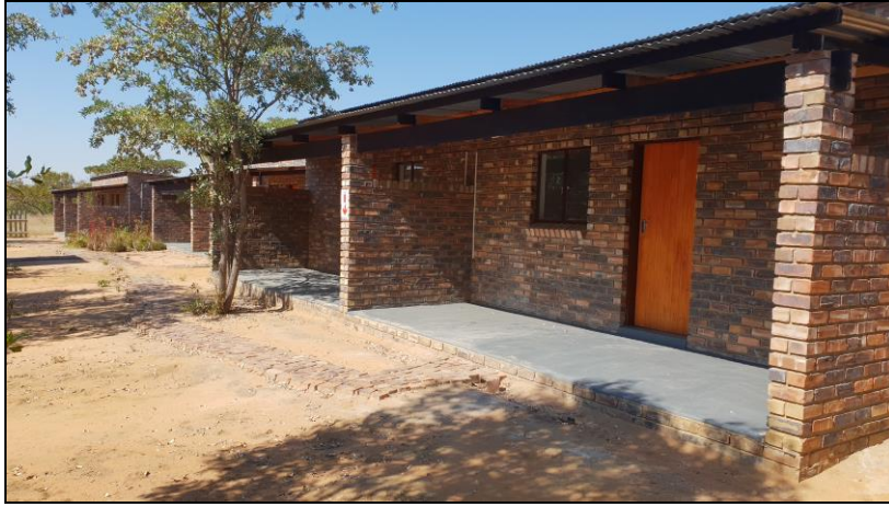
Figure 8: General view of the existing accommodation within the survey footprint (central section)
