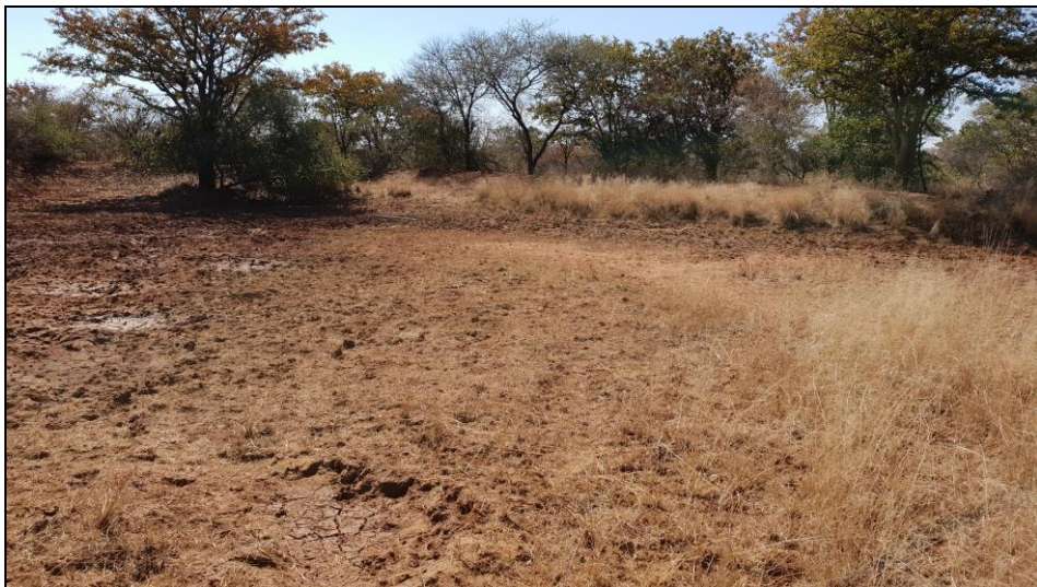
Figure 12: General view of the one of the small dams in the eastern section
