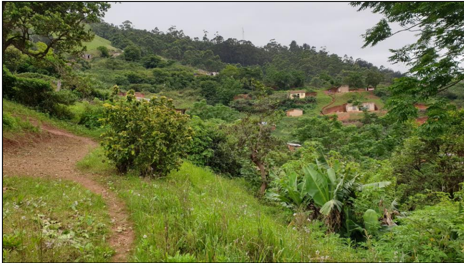
Figure 13: Existing infrastructure in Amatikwe Phase 2
