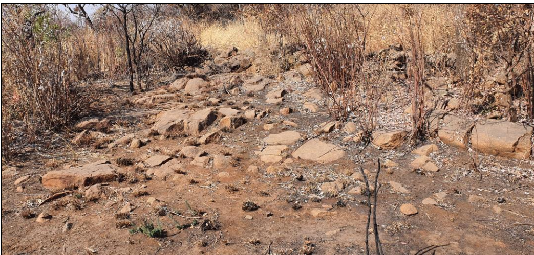
Figure 32: Some foundation walling in between the northern and southern section of the site
