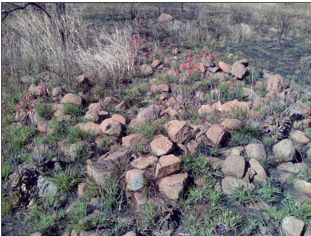
Figure 38: The foundation of the structure (no collapsed walling remained)
