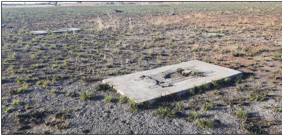
Figure 12: General view of the central section of the survey footprint (existing infrastructure)
