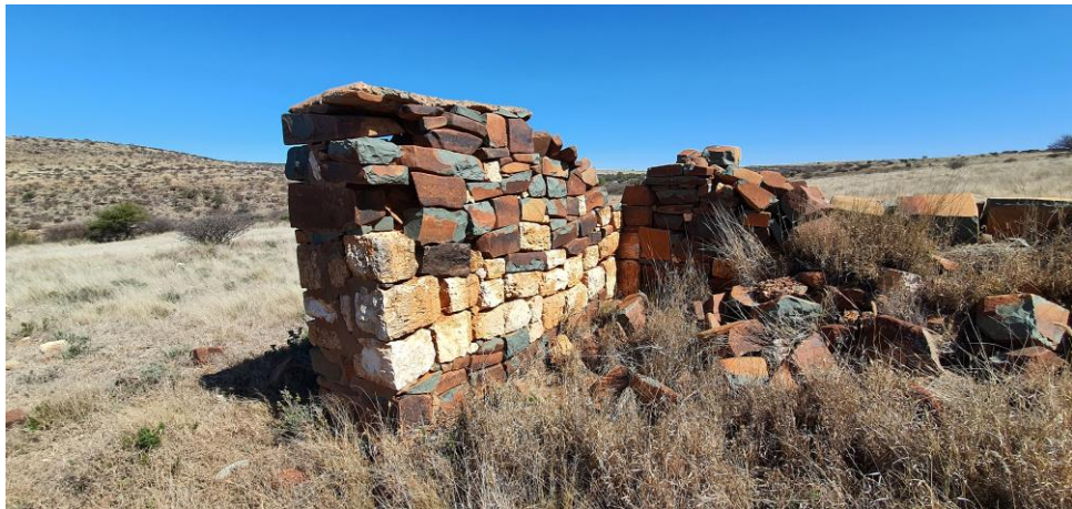
Figure 55: General view of the rondavel-like structure at this farm complex
