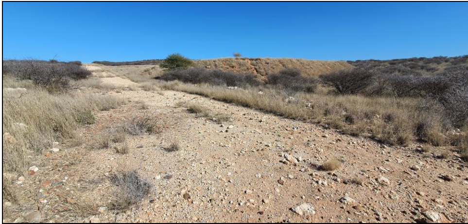
Figure 12: General view of the existing infrastructure within the survey footprint
