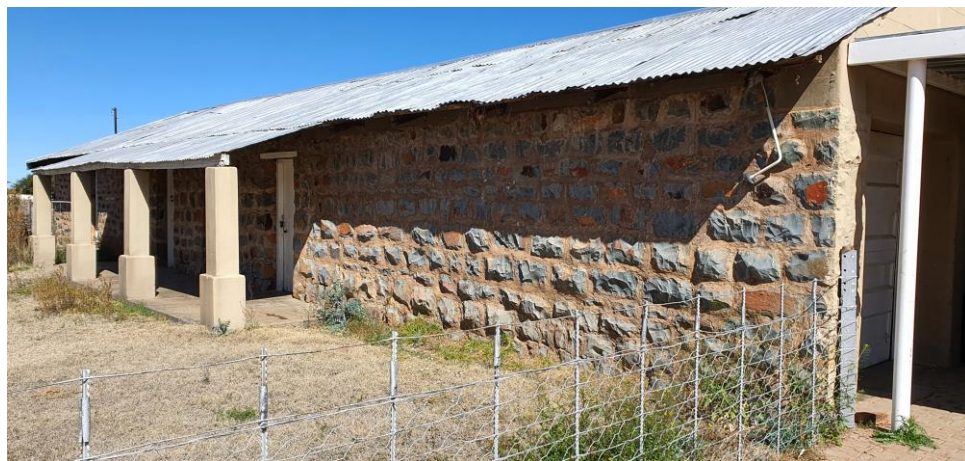
Figure 46: General view fo the farm shed built with dressed stones and corrugated iron roof
