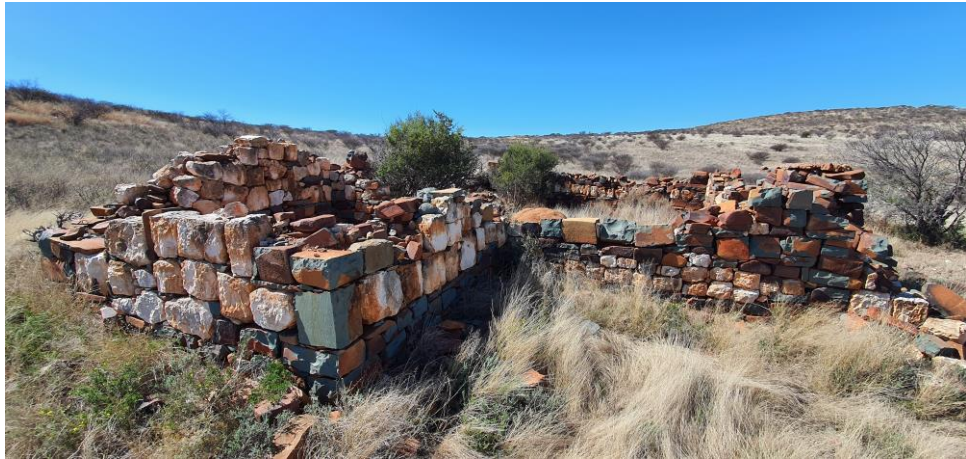
Figure 53: General view of the farmhouse complex
