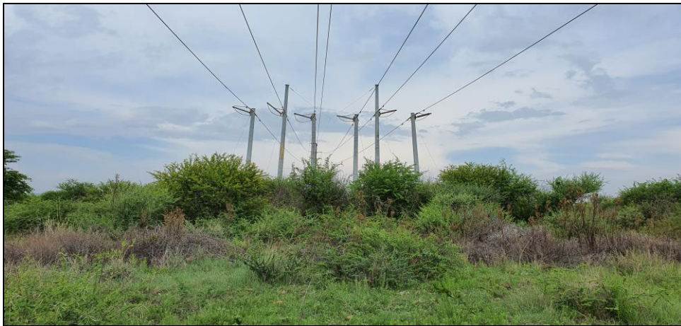
Figure 9: General view of the existing infrastructure
