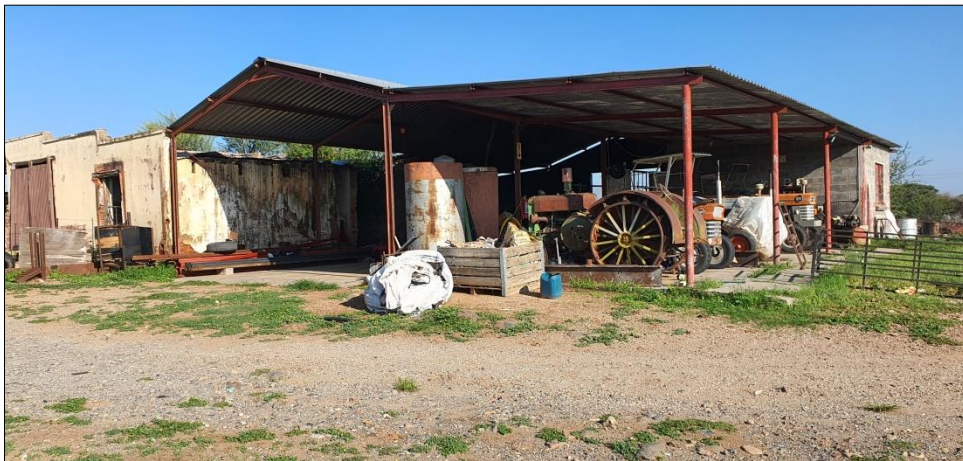
Figure 17: General view of the central south section (main outbuildings of the farm house on the farm Marktsdrift 3)
