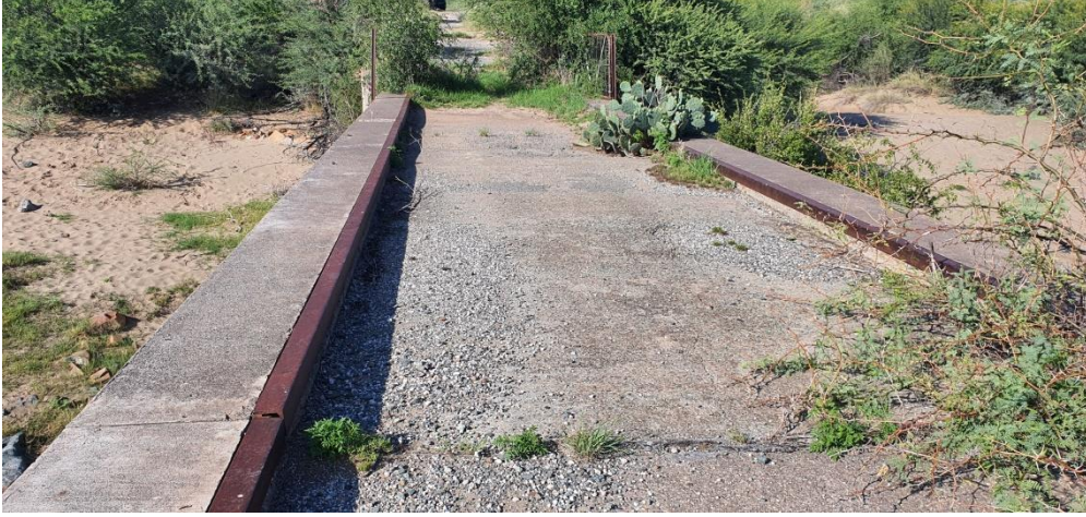
Figure 43: A general view of the bridge
