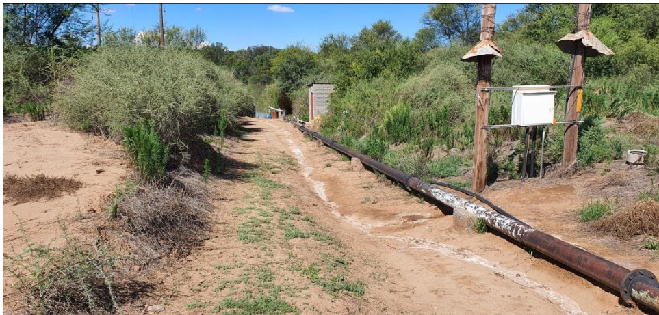
Figure 8: General view of the southern section (existing infrastructure) of the survey footprint
