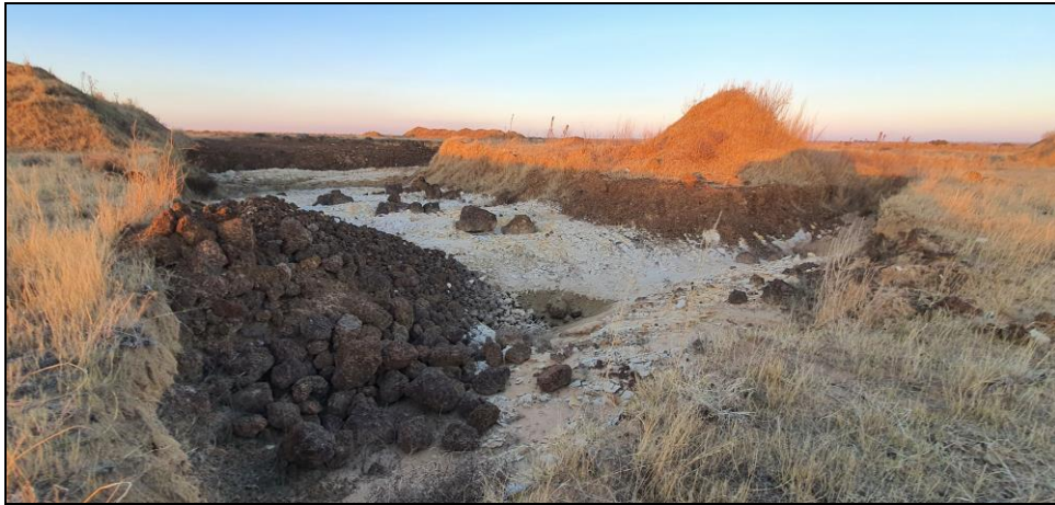
Figure 13: General view of the southern section of the survey footprint (old mining activities)
