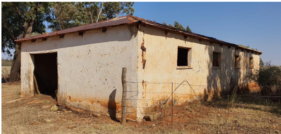
Figure 51: General view of the shed associated with the main farmhouse
