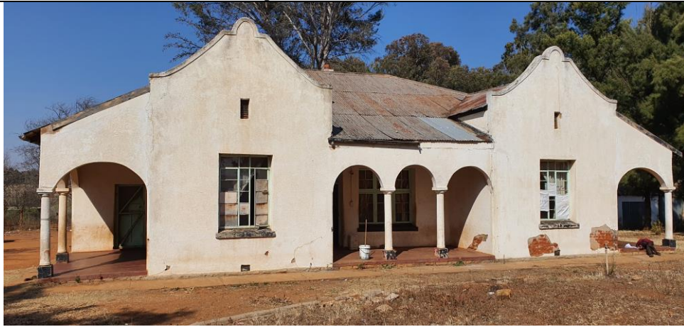
Figure 49: General view of the northern façade of the historical farm house
