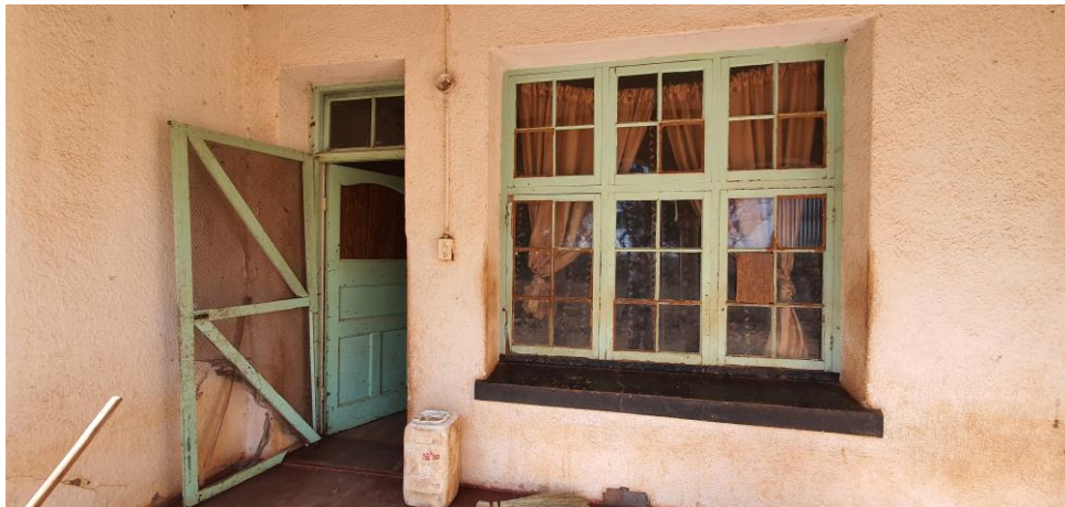
Figure 50: General view of the front door and window (wooden frames)
