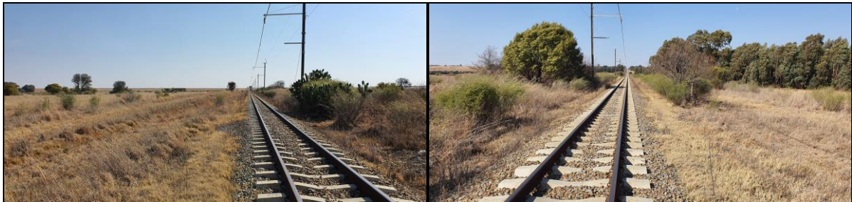
Figure 22: General view of the northern section of the survey footprint (railway line)
