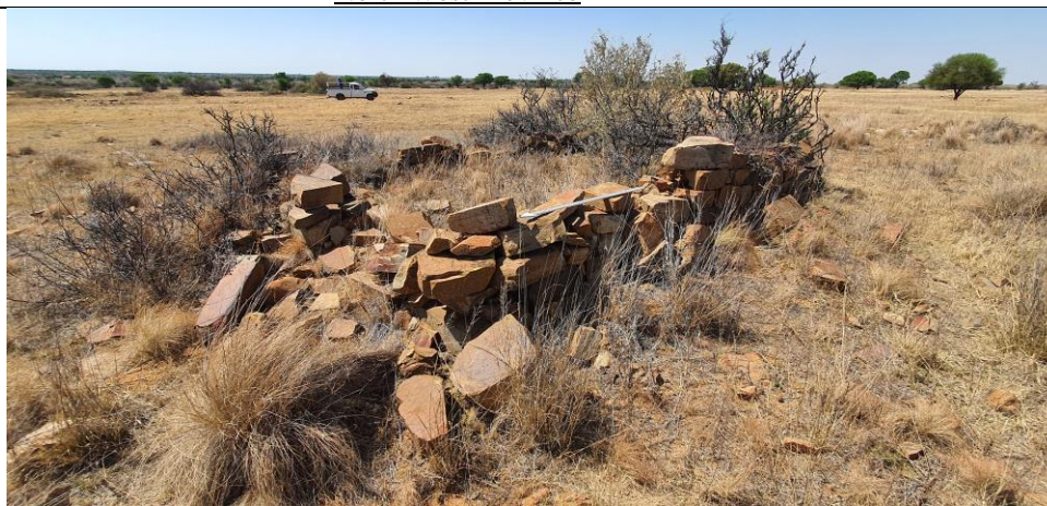
Figure 36: General view of the western section of the historical structure
