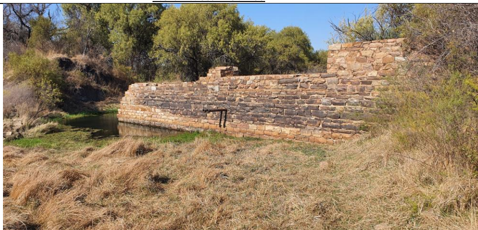
Figure 39: General view of the historical dam wall
