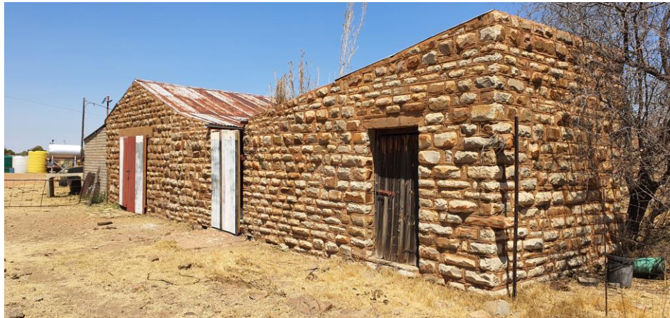
Figure 42: General view of the dressed stone sheds
