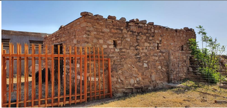
Figure 41: General view of the block house
