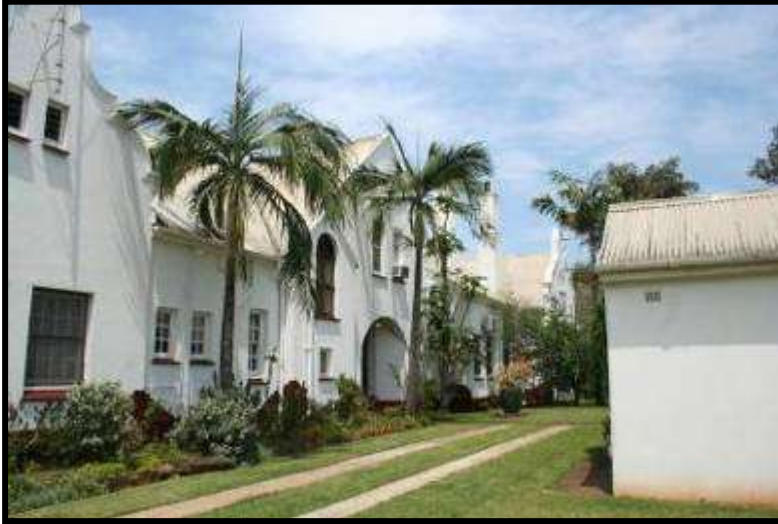
Fig 4.3: Rear view of Highfield Country House (photo: supplied)
