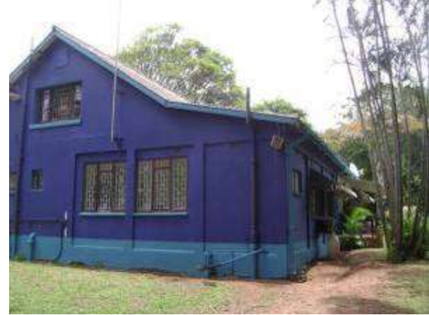
Fig 3.2 Main house from east
