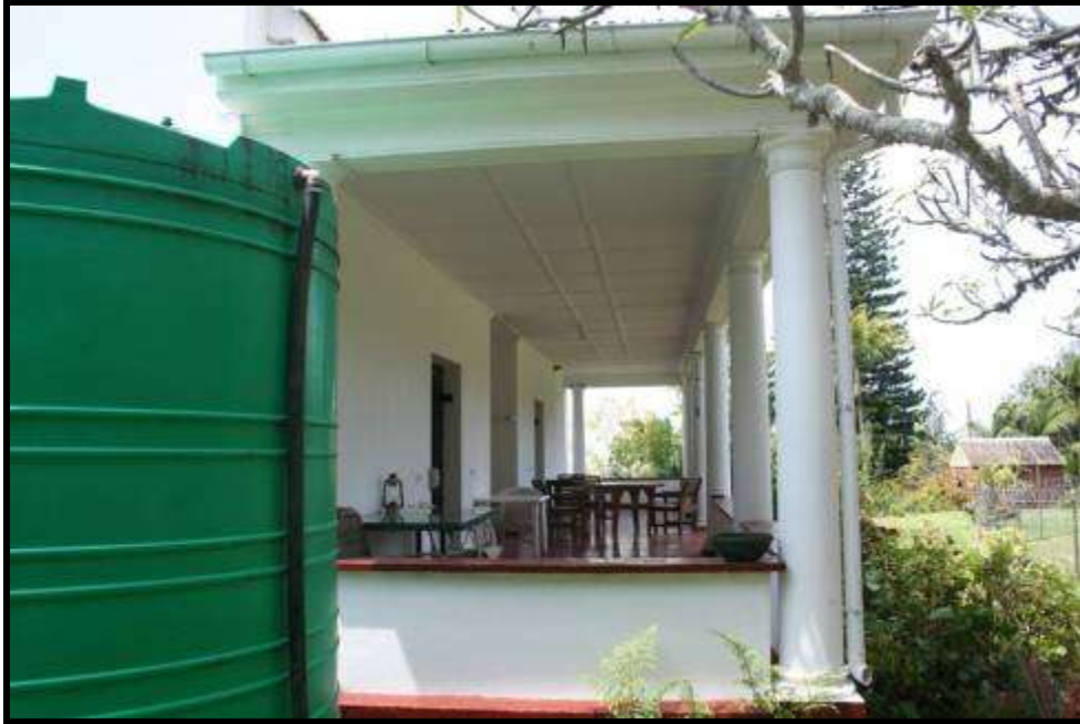
Fig 17: Veranda of main structure- Highland House (photo: supplied)
