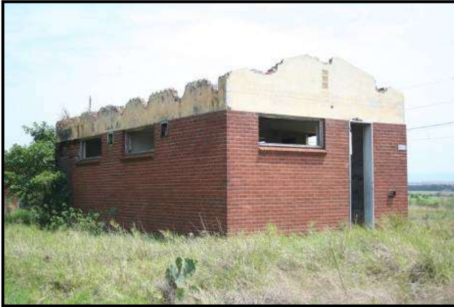
FIG 6: SHOWING REMAINS OF STATION BUILDING (PHOTO: SUPPLIED)
