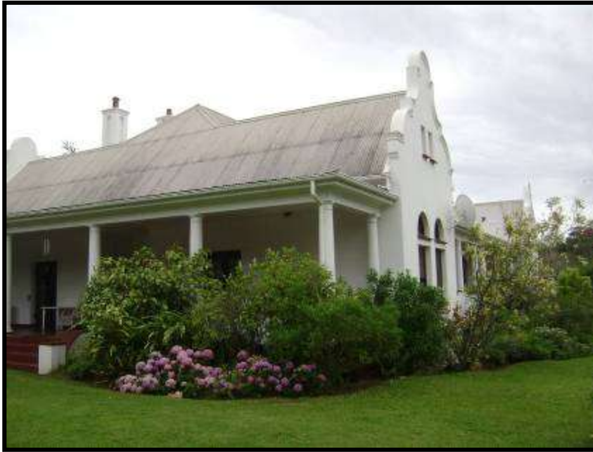
Fig 4.5: view of the south west corner from the garden
