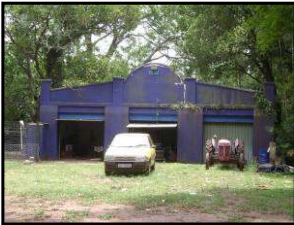
Fig 3.13: garage/ shed constructed in 1921.
