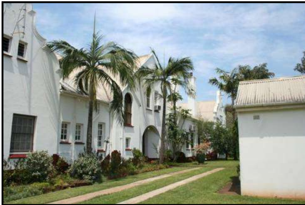
FIG 16: REAR VIEW OF HIGHFIELD COUNTRY HOUSE (PHOTO: SUPPLIED)
