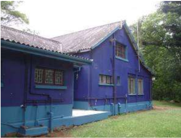
Fig 3.1 Main house east elevation
