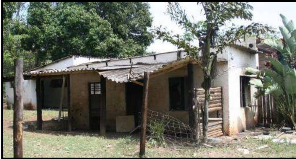
FIG 20: HOUSE 2 LABOURERS COTTAGE (PHOTO: SUPPLIED)
