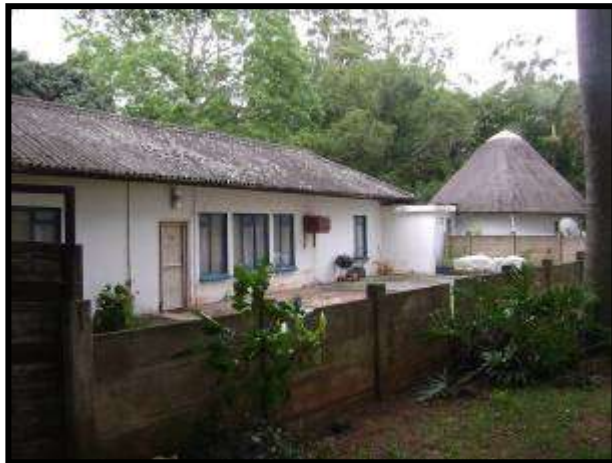
Fig 3.17: second dwelling, 1950's 1960's conventional materials under corrugated asbestos sheeting
