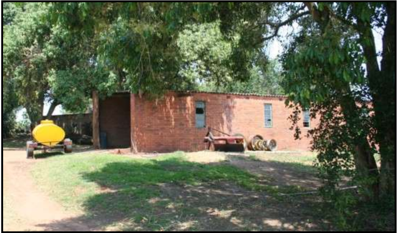
FIG 27: OUTBUILDING (PHOTO: SUPPLIED)
