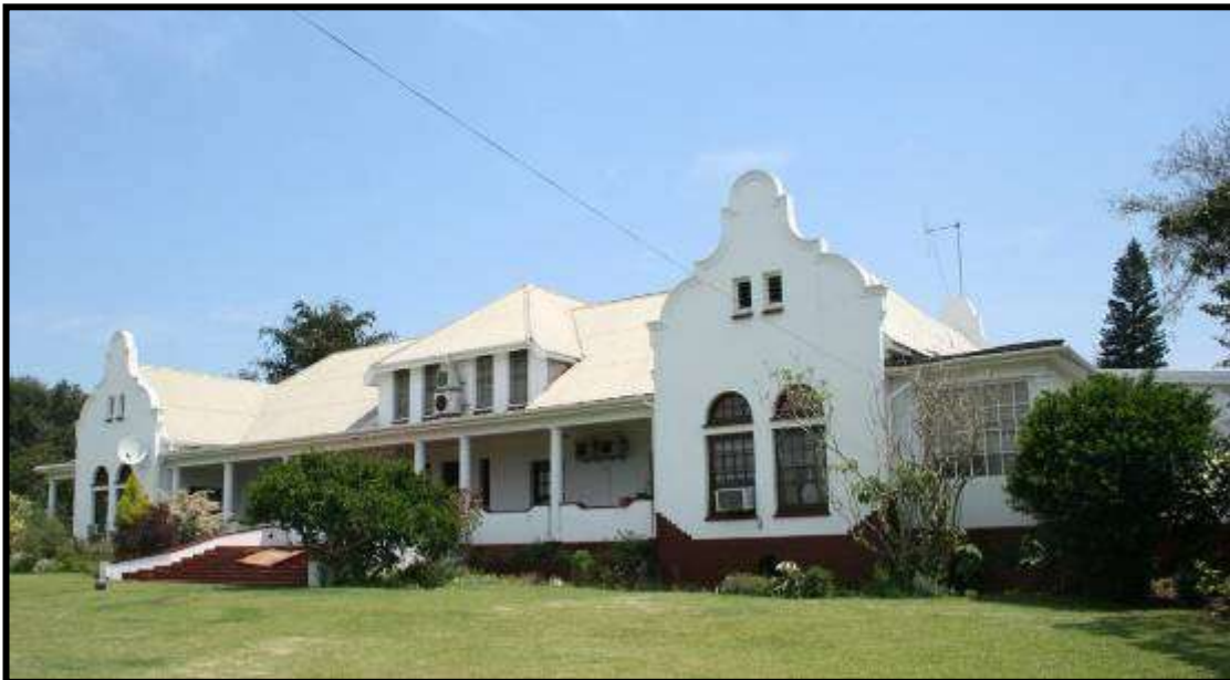
FIG 14: SHOWING FRONT ELEVATION OF HIGHFIELD COUNTRY HOUSE (PHOTO: SUPPLIED)
