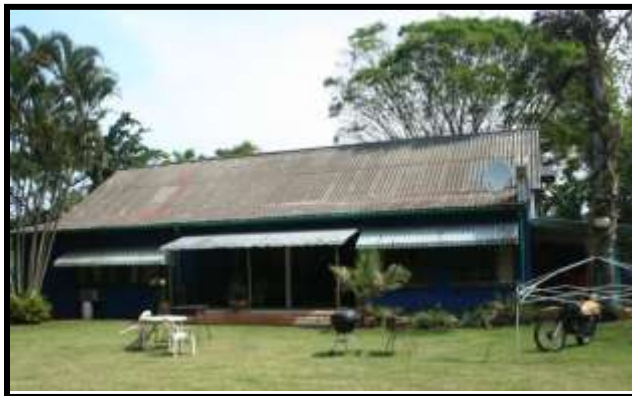
Fig 3.3 north east elevation (author 2010)
