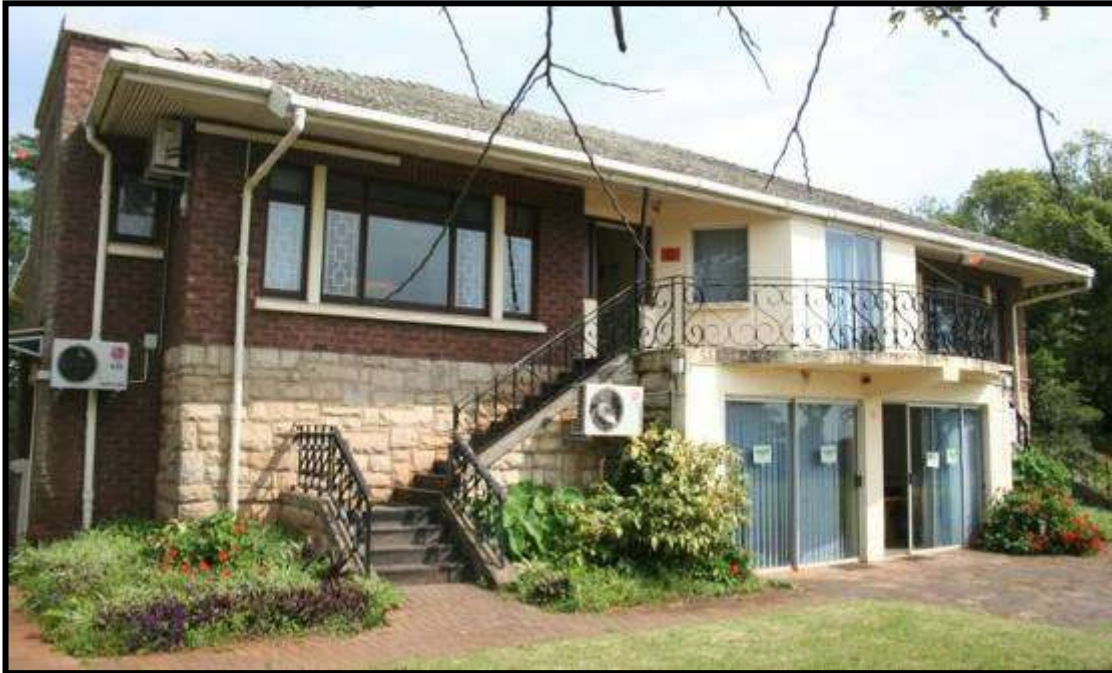
FIG 2: AFFECTED STRUCTURE ON LOT 91 UMLALAZI (PHOTO: SUPPLIED)
