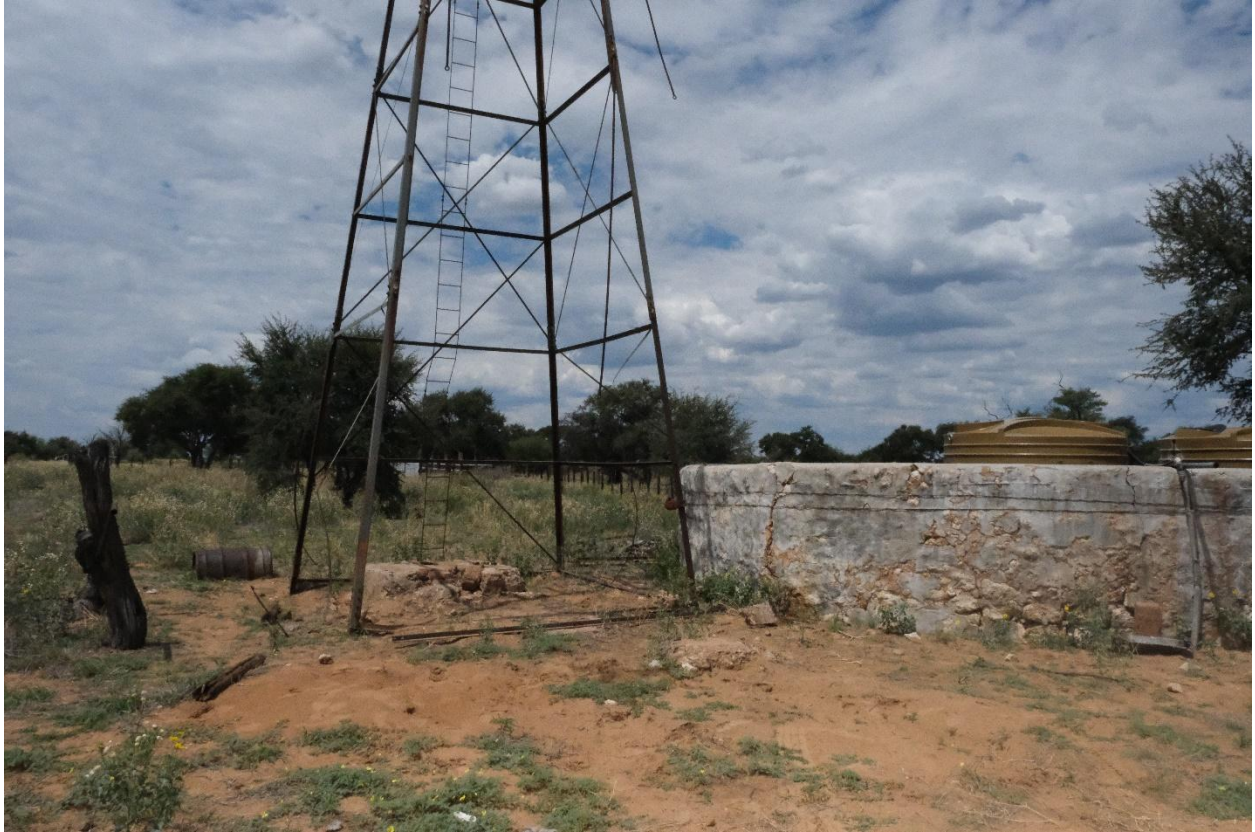
Figure 11: Windmills and water storage concrete on Portion 59 of Farm 703 (Photo by Pulafel 4D 2023).
