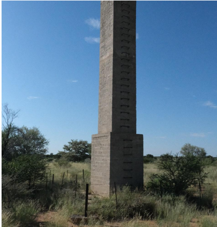
Figure 8: Possible Historical structures in Portion 116 of Farm 703. Photo by Pulafel 4D (2023).
