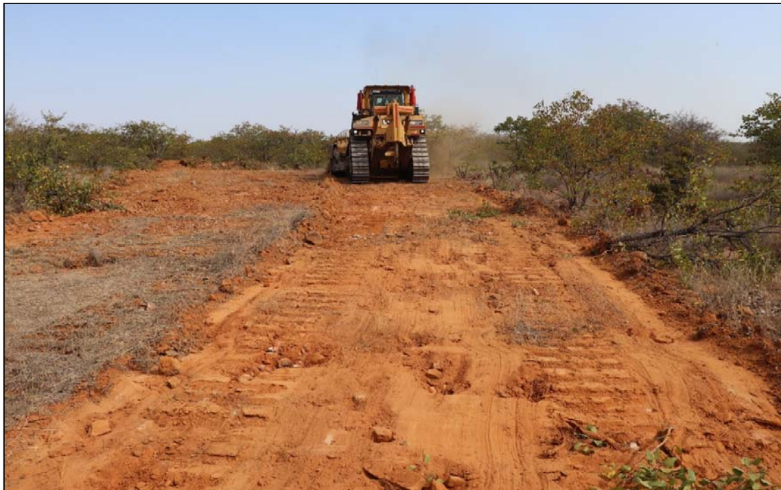
Figure 6: Dozer clearing the site
