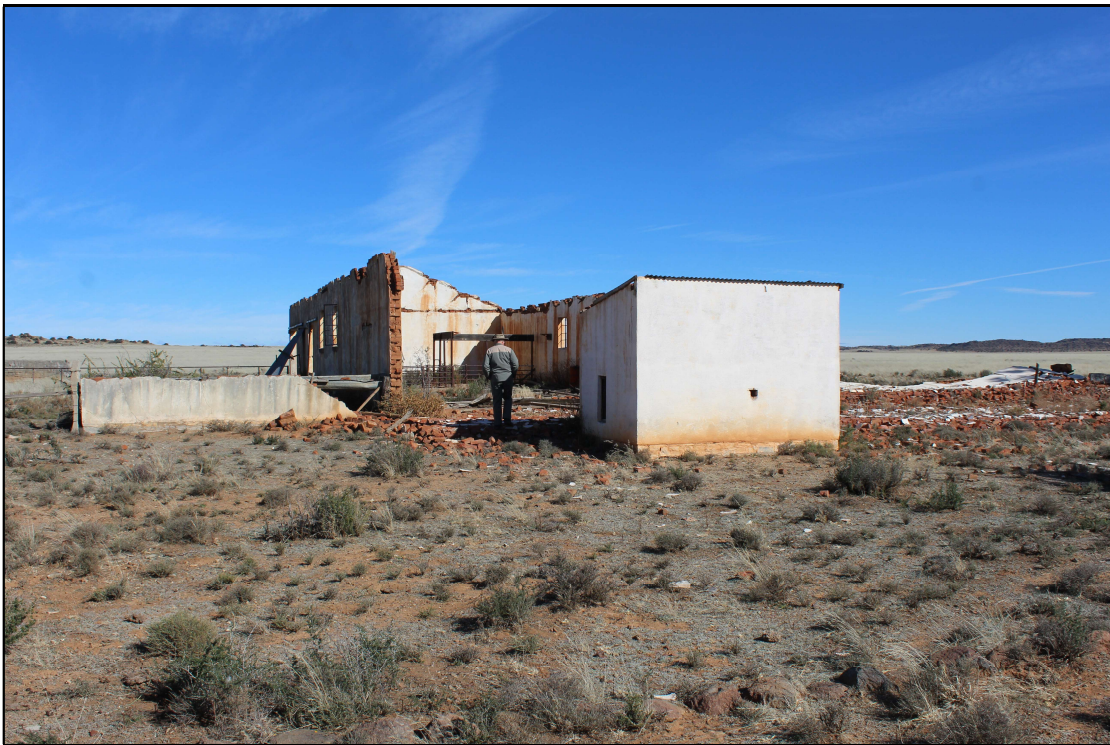
Figure 3: Associated infrastructures some dilapidated noted adjacent to the historical building
