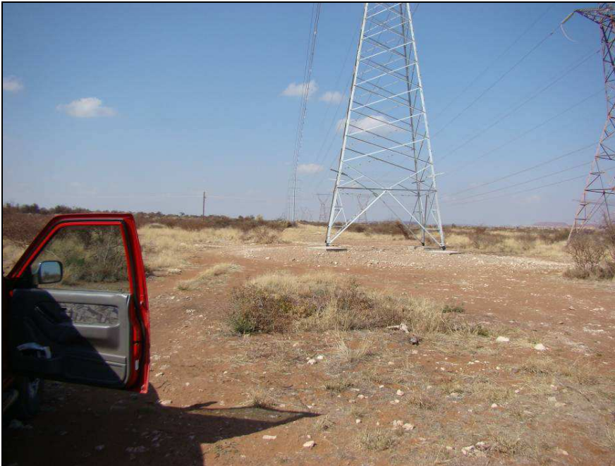
Fig.13 Pylon K5 outside Kathu.
