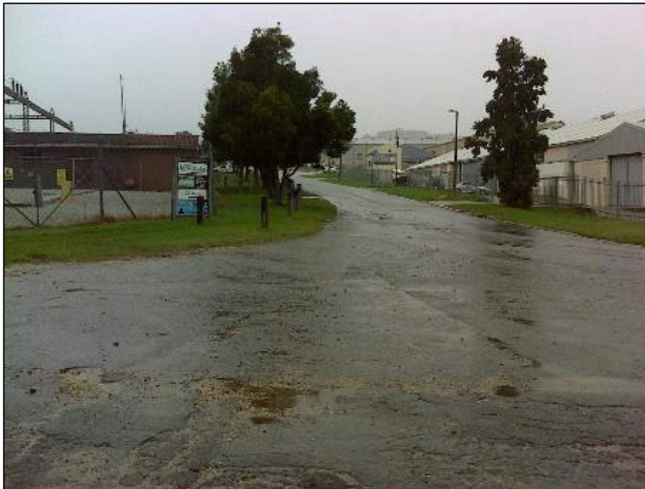
Figure 4. View of the built-up Knysna Industrial area at the corner of Waenhout Avenue and Boswerker Street.
