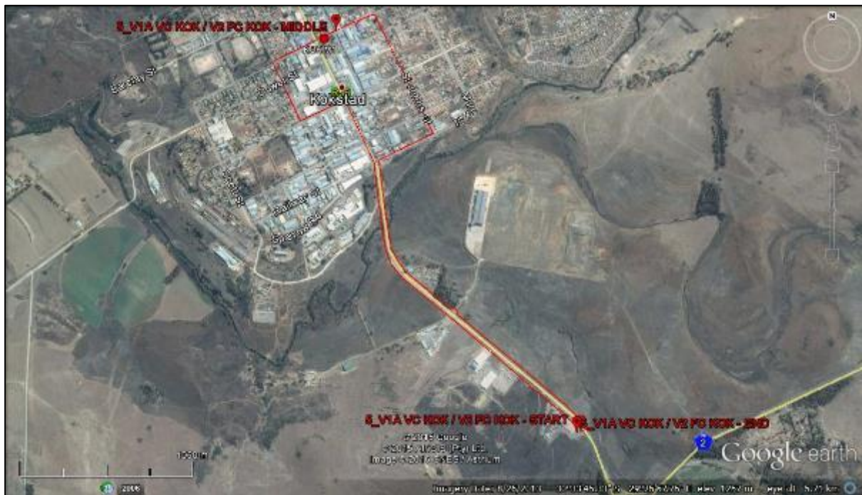
Figure 53. Aerial view of the deviation route for Repeater Site V1A VC KOK/V2 FC KOK running through the town of Kokstad.
