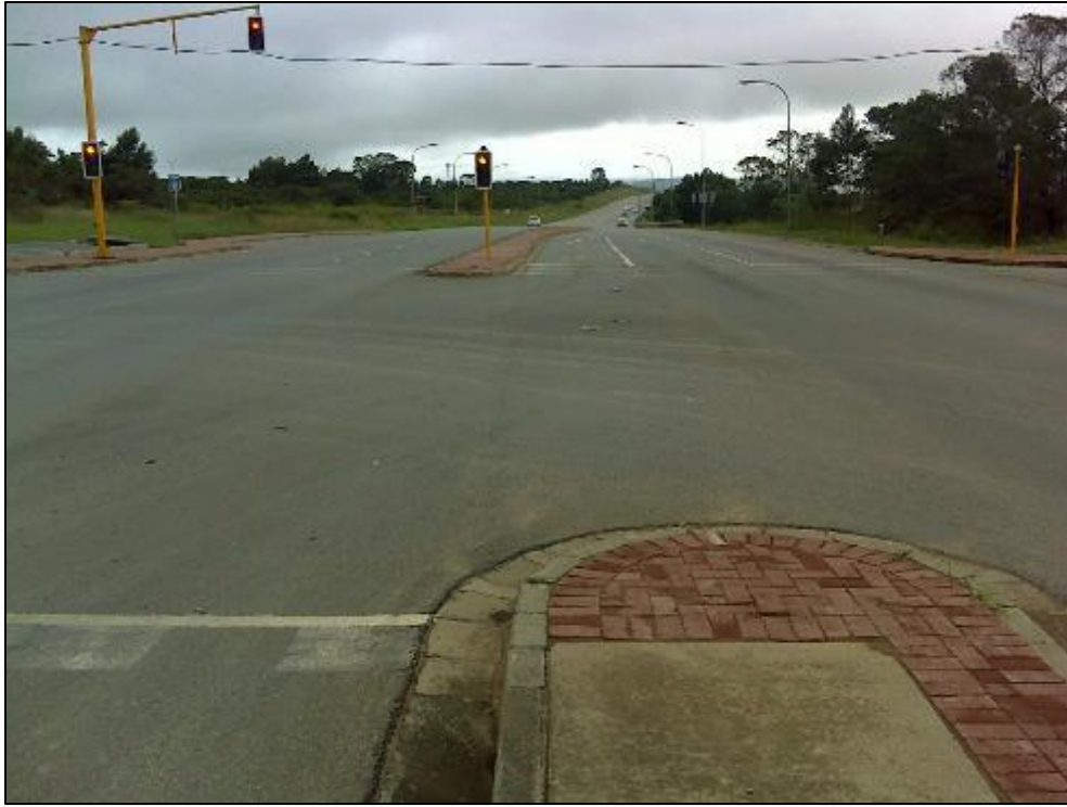
Figure 32. View of Maitland Road facing north towards Bhisho.
