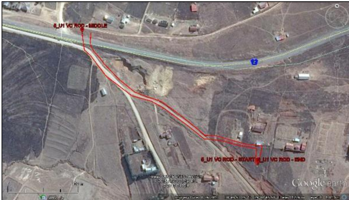
Figure 51. Aerial view of the deviation route for Repeater Site U1 VC ROD situated off the N2 national road between Mount Frere and Mount Ayliff.
