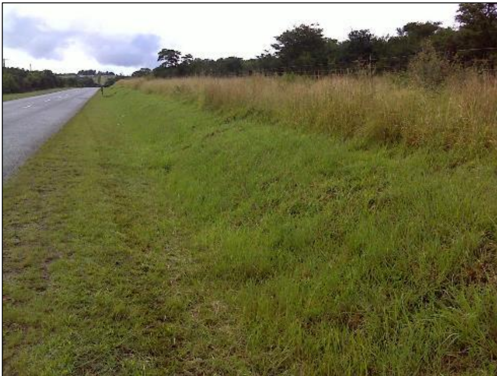
Figure 37. View of the road reserve between the N2 and Komga along the R63.
