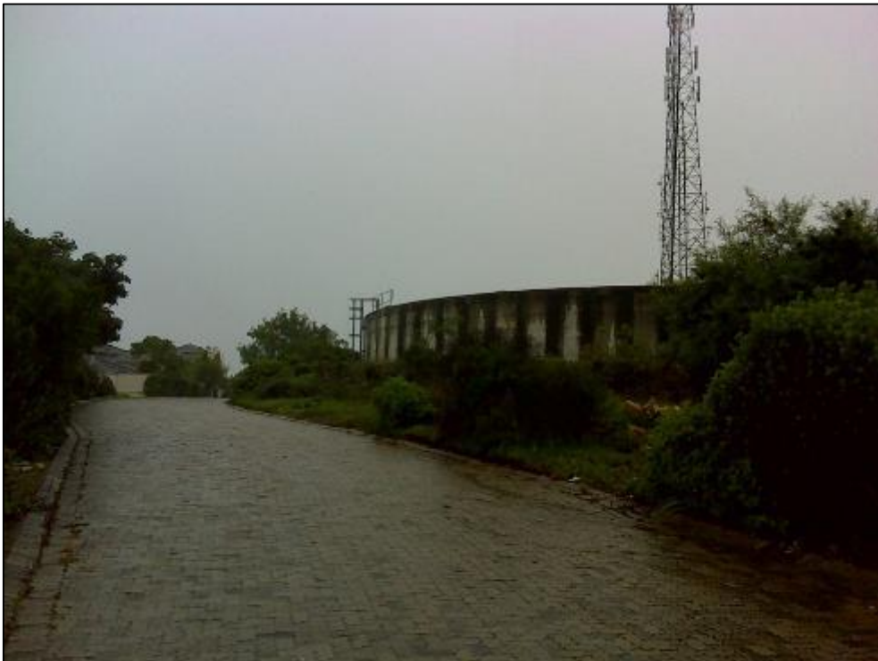
Figure 7. View of the developed resort / residential area showing the repeater tower and one of the two reservoirs situated within the complex.
