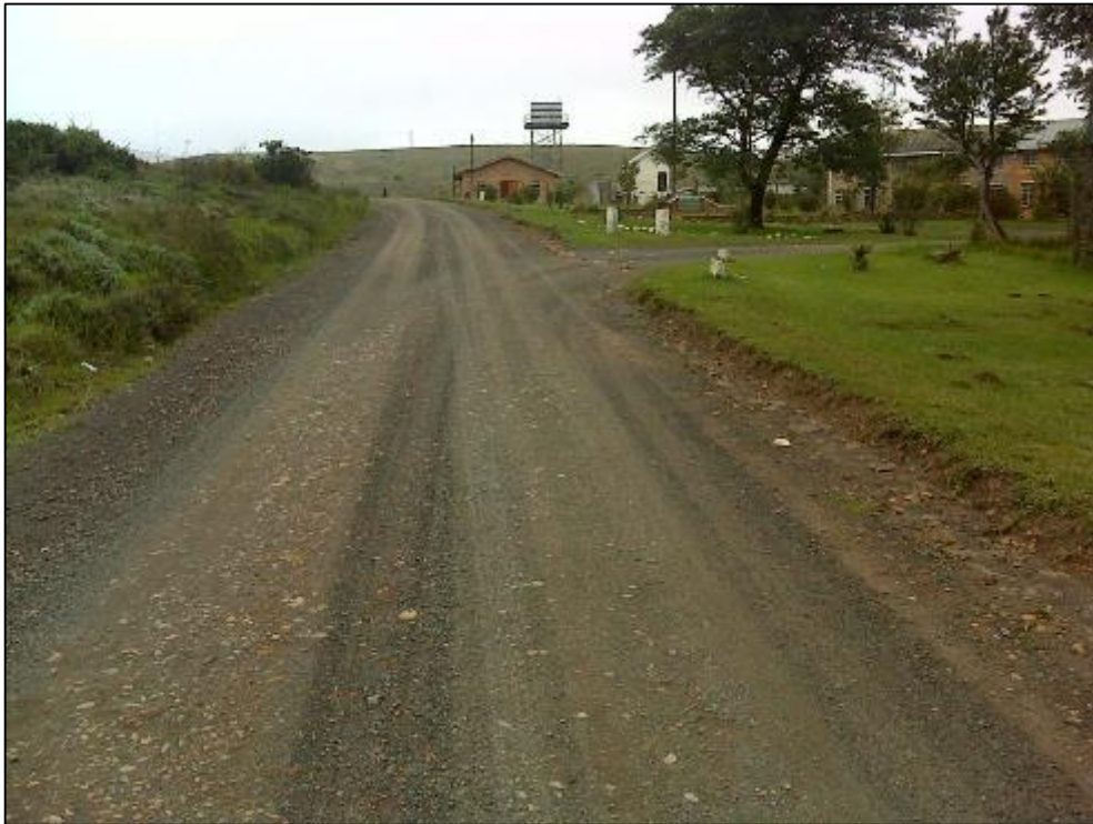
Figure 23. View of the deviation route at the Grahamstown Water Works.
