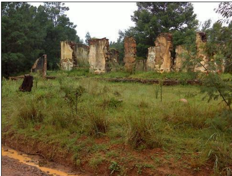
Figure 14. Building ruins situated HUM BE1.
