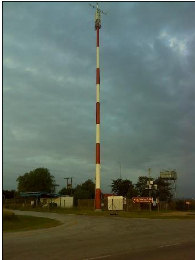
Figure 20. View of the repeater site situated at the Kinkelbos Traffic Calming Centre.
