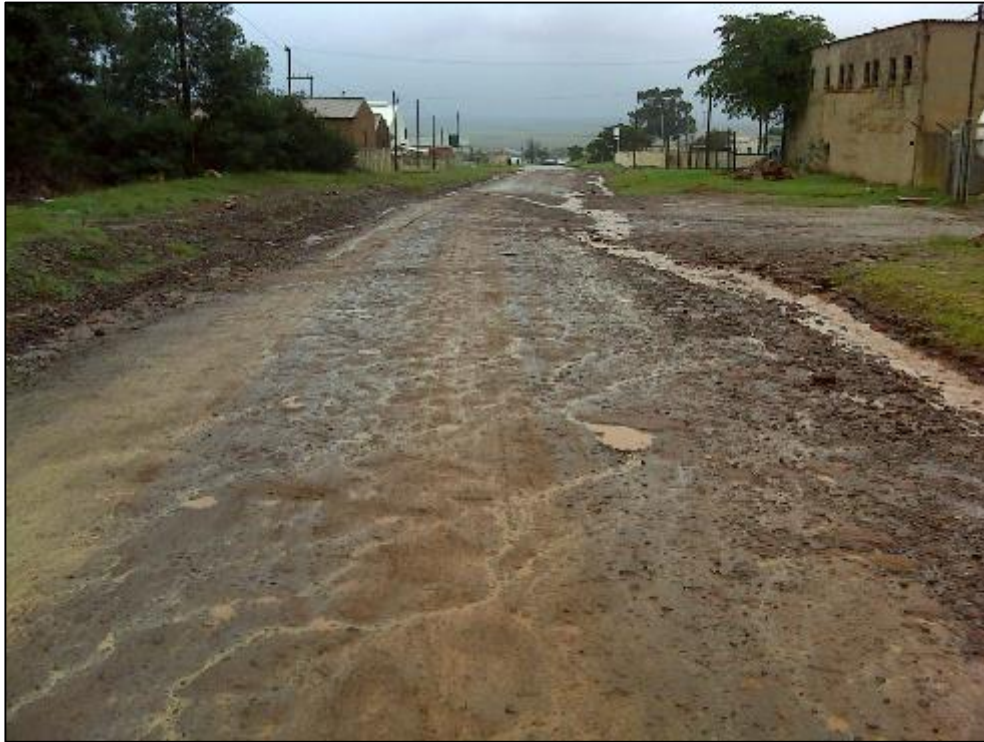
Figure 12. Street view of Humansdorp's Industrial area.
