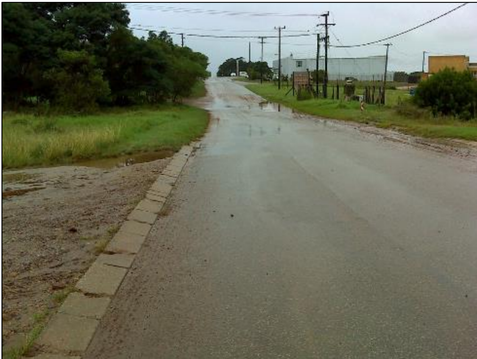
Figure 13. Street view of Humansdorp's built-up Industrial area.
