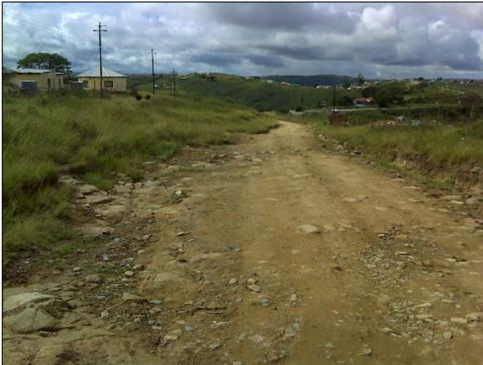
Figure 41. View of the road leading to the repeater site showing the dense vegetation cover, power lines and fences.
