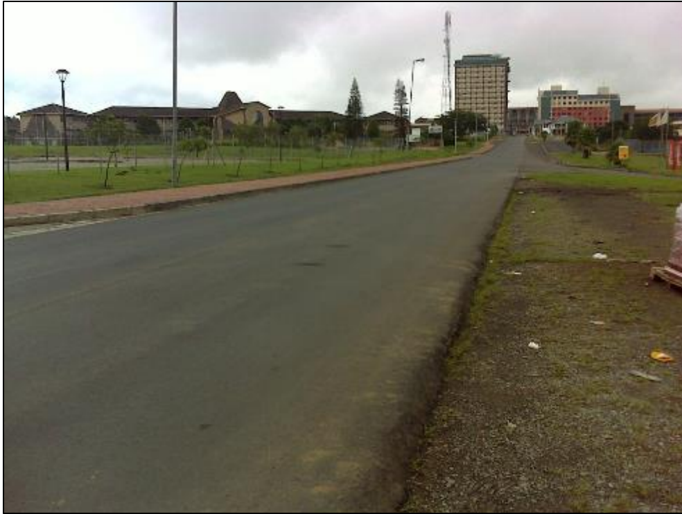
Figure 34. View of Independence Avenue facing north towards Bhisho central.
