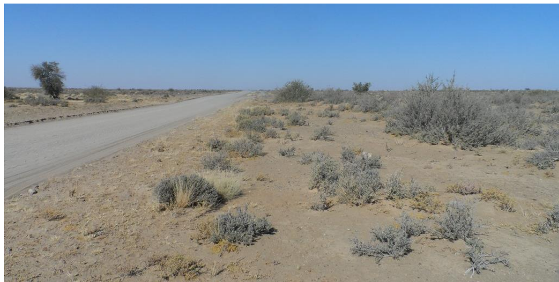
Figure 19: Typical view of pipeline route between Philandersbron and Rietfontein
