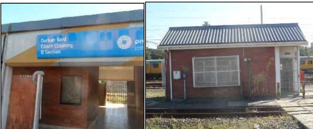
Figure 10- Coach cleaning facilities and shunters resting rooms
