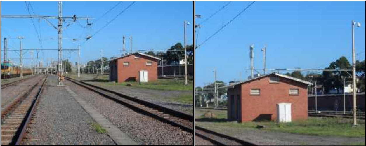
Figure 25- Control cabin point - shunters
