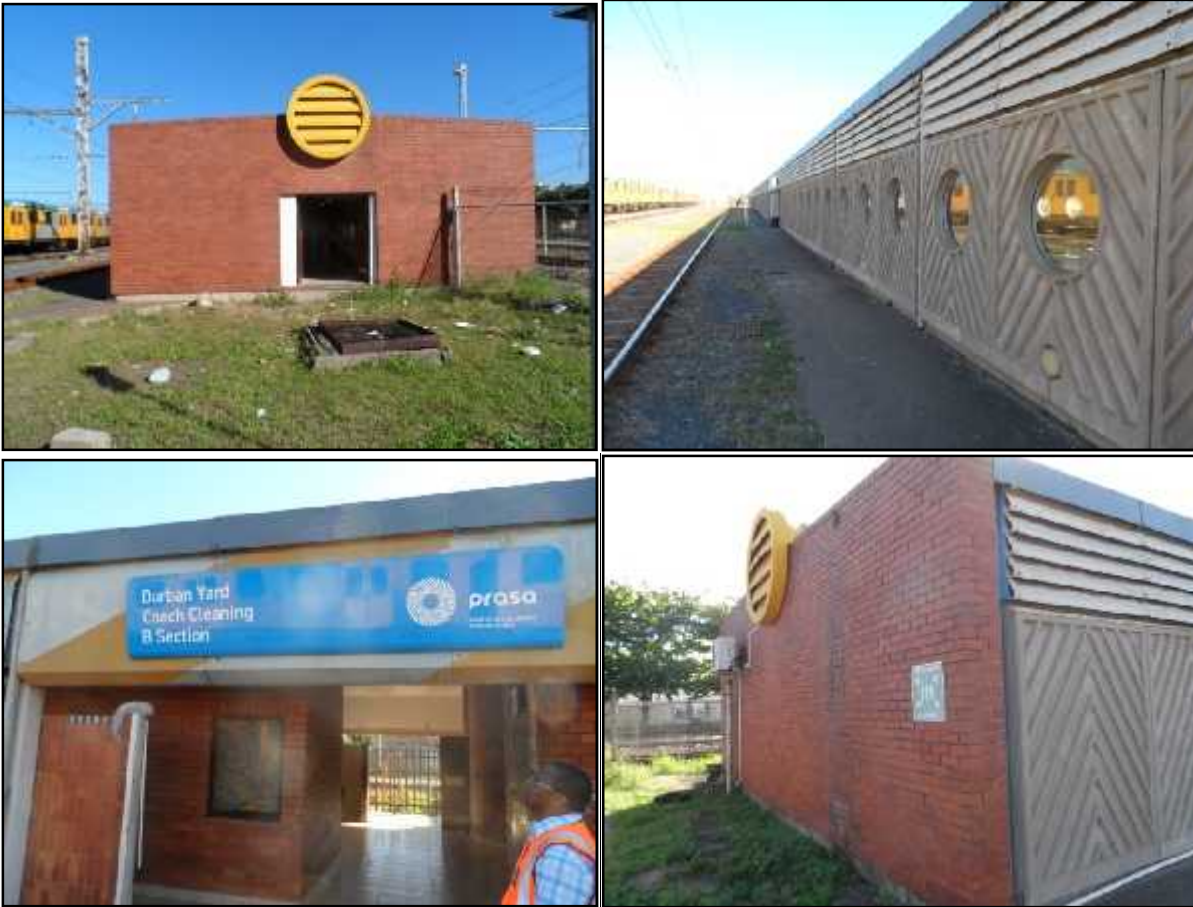
Figure 20- Durban Yard PRASA coach cleaning building
