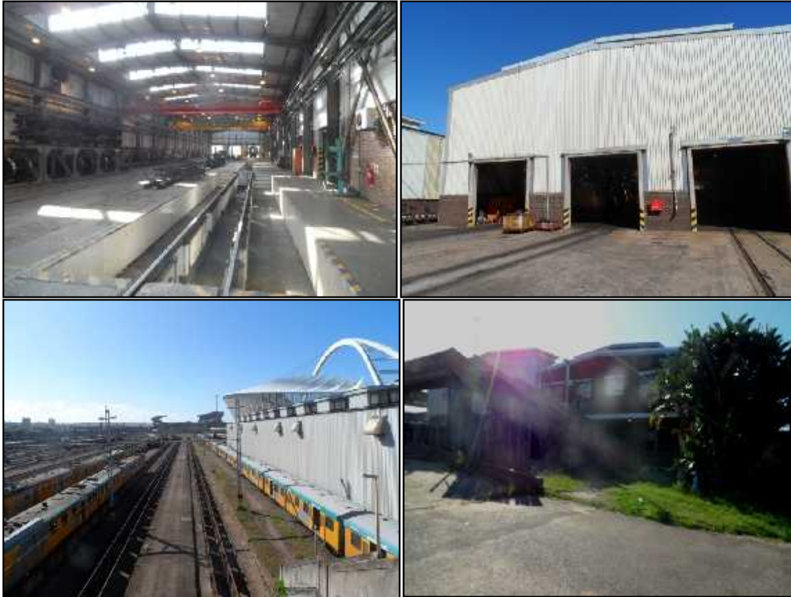
Figure 14- Train lifting shop shed (internal & external views) and offices attached to the lifting shop.
