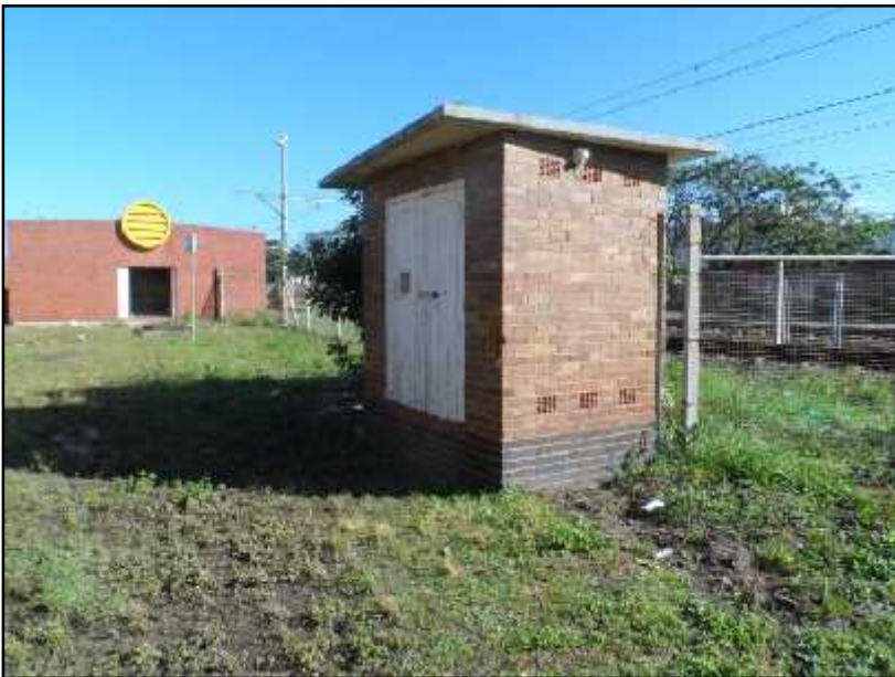
Figure 19- control cabin point
