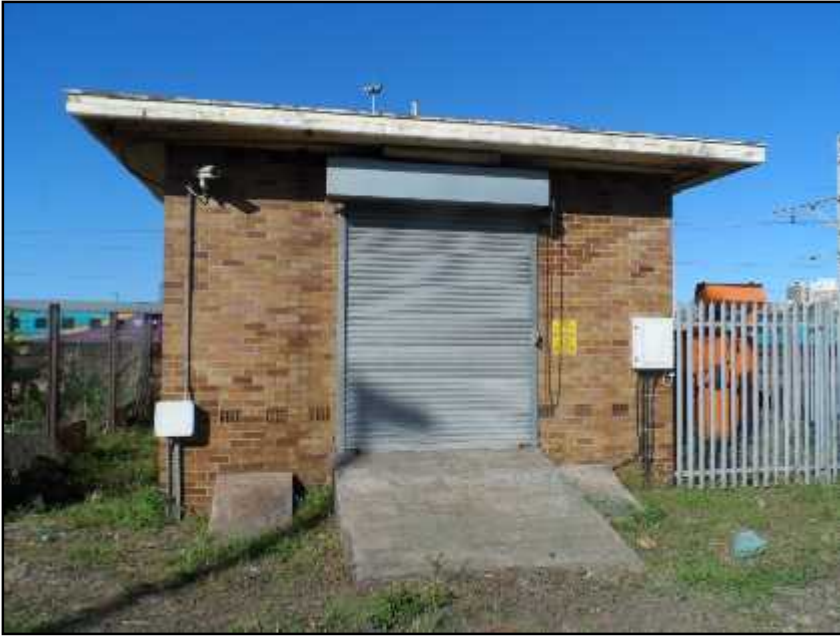
Figure 27- old storage structure
