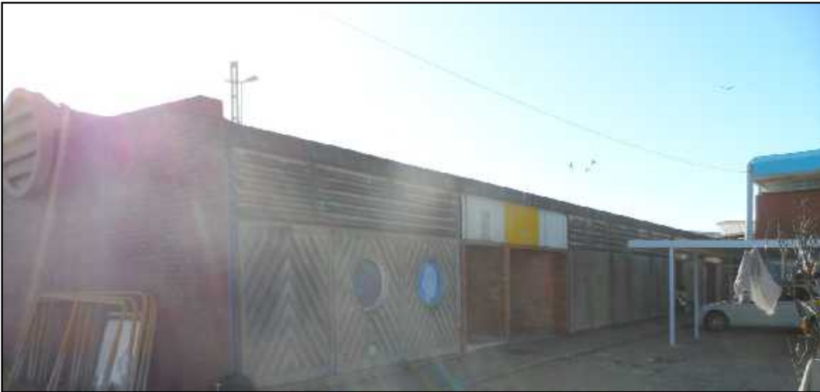
Figure 30- Electric power generating structure
