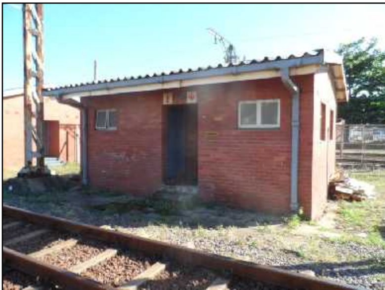
Figure 17- Train drivers/shunters ablution facilities
