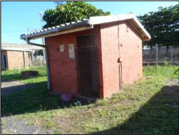
Figure 21 - Control cabin point- shunters
