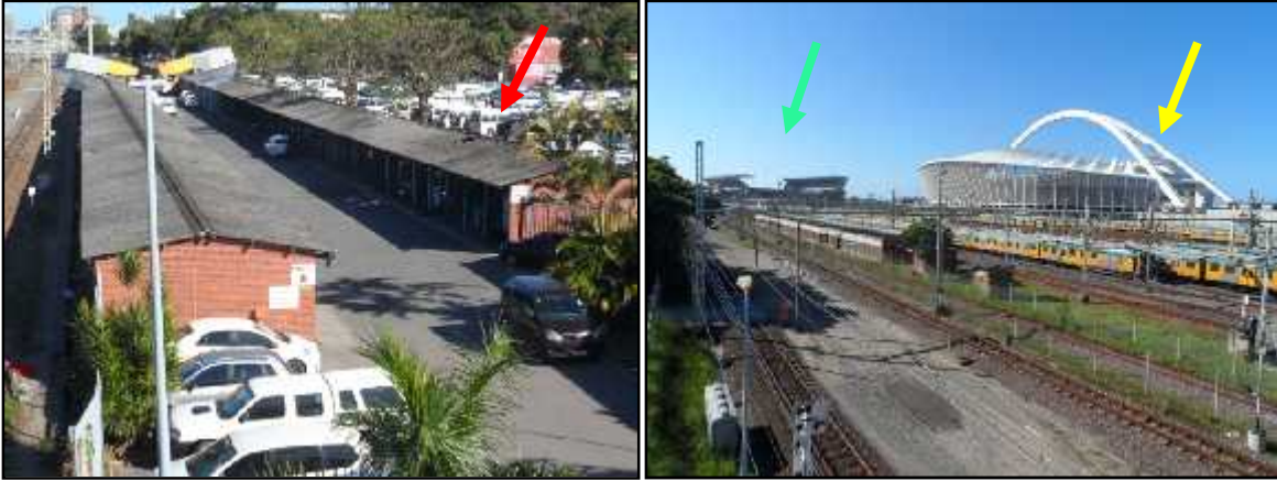
Figure 8- Surrounding infrastructure - A taxi rank behind Durban PRASA depot parking area (red arrow), Kings Park Stadium (green arrow) and Moses Mabida Stadium (yellow arrow).
