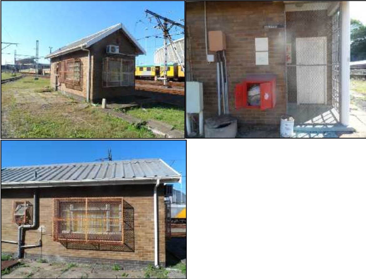
Figure 16- Control cabin point
