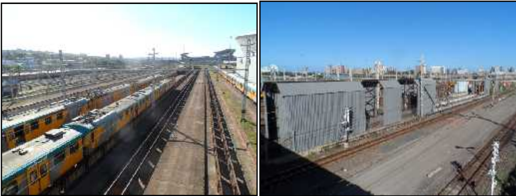
Figure 9 - Rail infrastructure (tracks and coaches) and external washer.
