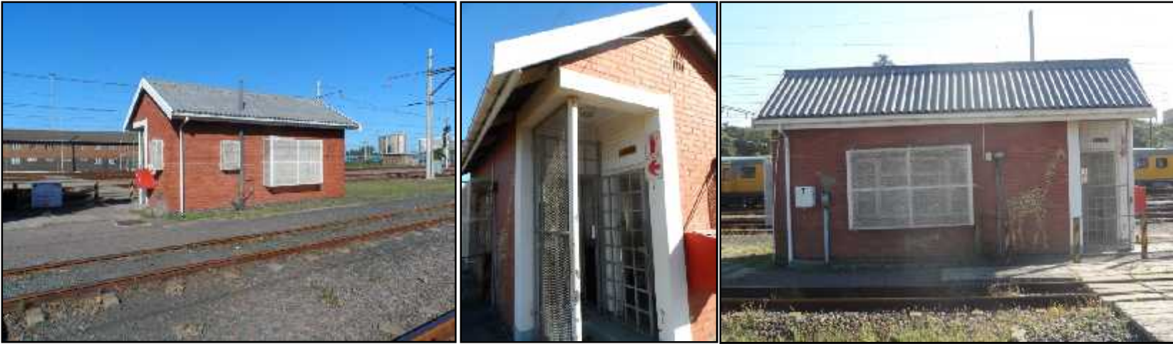
Figure 26 - modernised and decorated control point cabin
