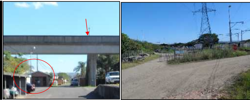
Figure 10 - Access road to site (security check point (red circle) & overhead bridge - red arrow) and a unpaved truck road (left)
