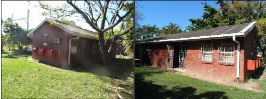
Figure 16 -shunters/drivers office and rest room
