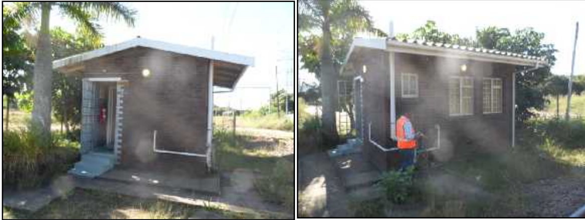
Figure 18- Shunters/coach operations control cabin
